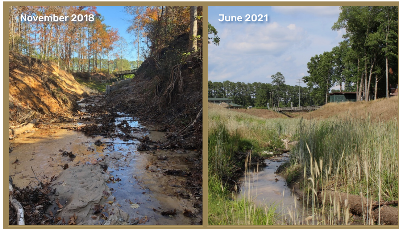
Figure 5.33 Before and after, Methodist University stream restoration (McAdams)
