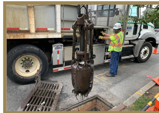
Figure 5.24 Cleaning dirty catch basins in the Big Apple (NYC Environmental Protection)
