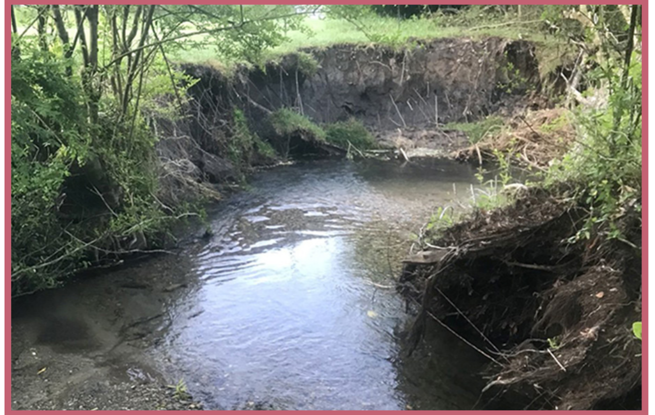
Figure 2.12 Streambank erosion caused by hydrologic impacts (Clemson University)
