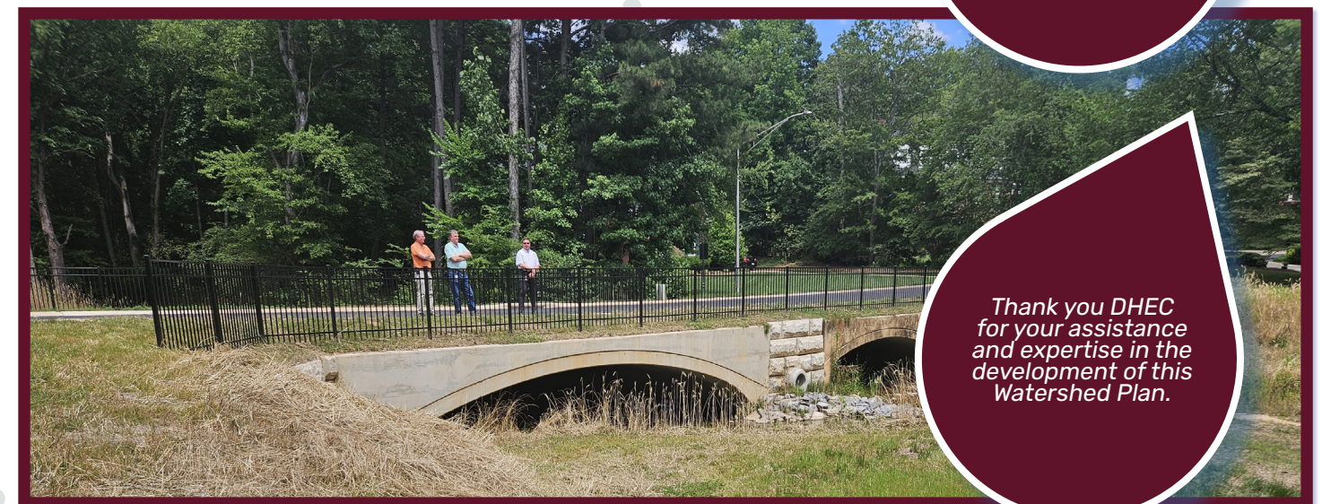
Figure 2. Photo of completed stream restoration (McAdams)
