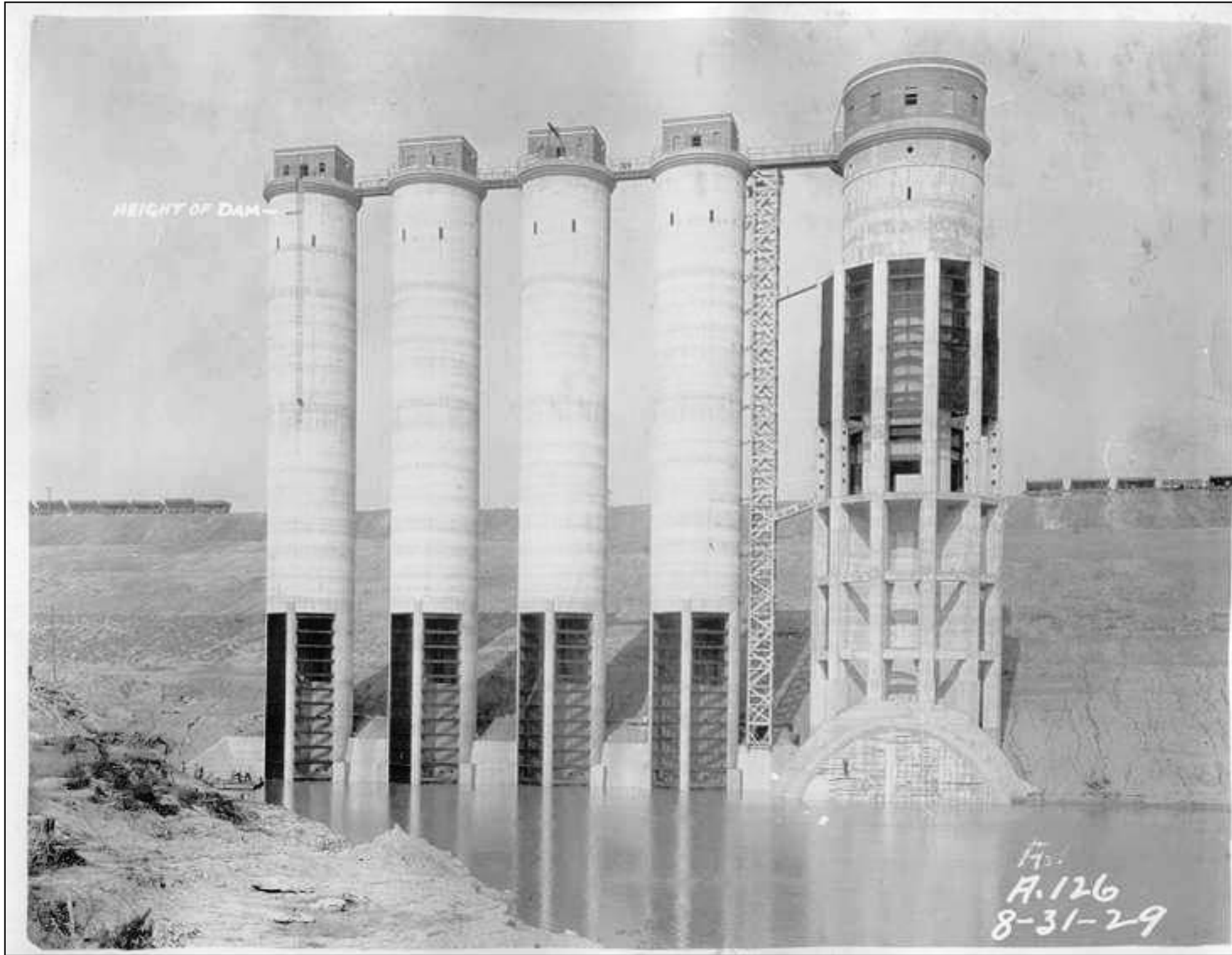
Intake Towers, August 1929
