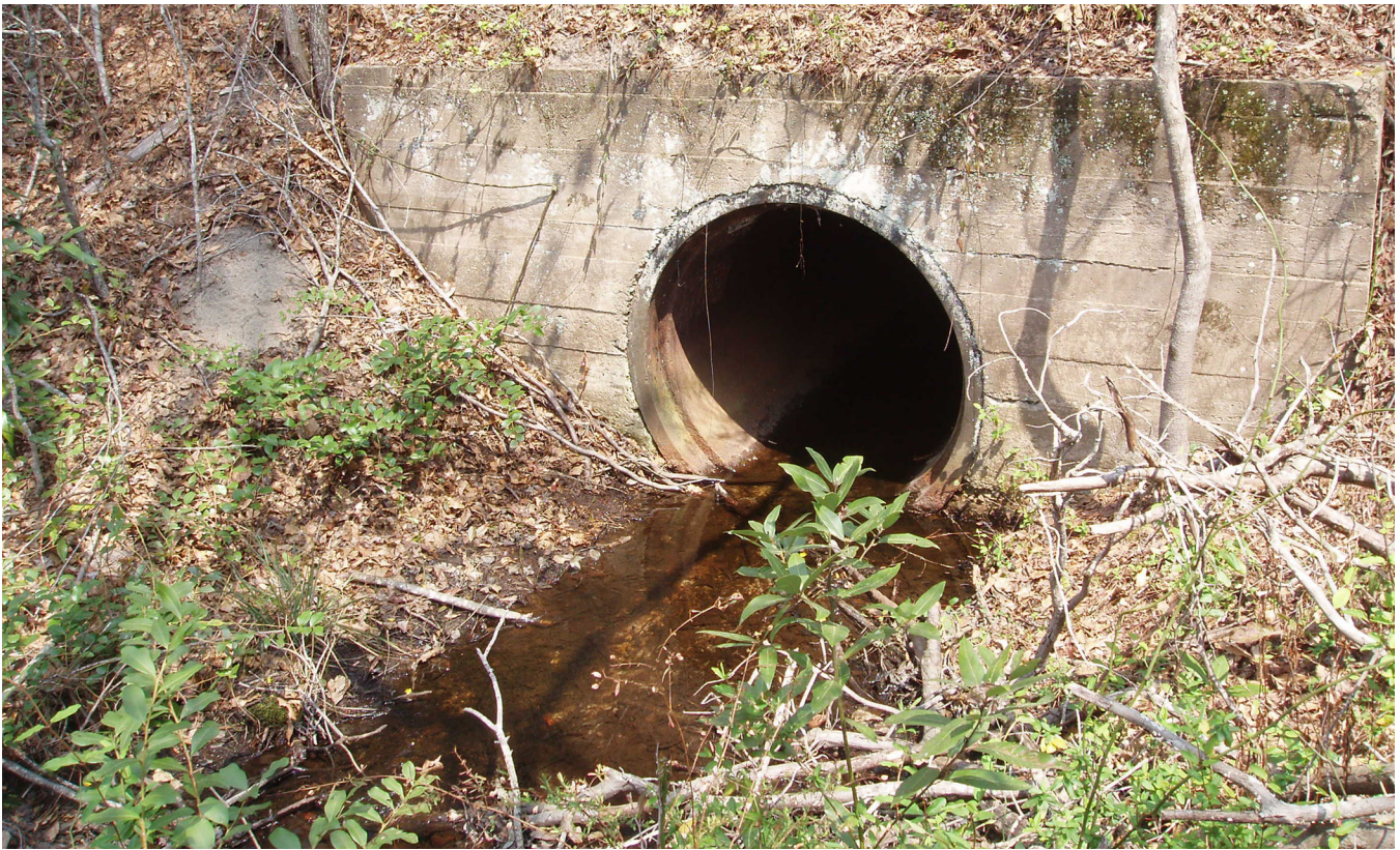
Figure 3. Outlet culvert draining the WPB and DPB ditches.
