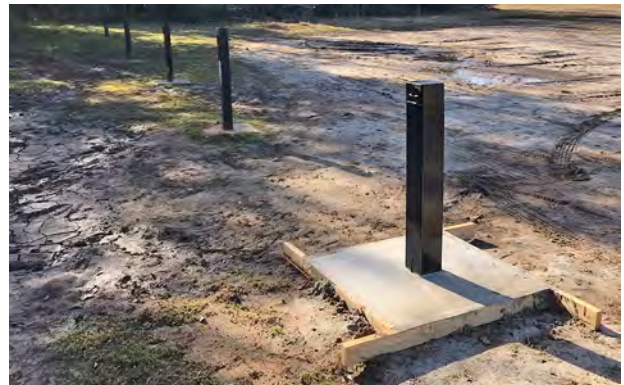
Figure 28. The new monitoring well CAL-0215, screened in the McQueen Branch aquifer, at the Creston cluster site. In the background are the four monitoring wells installed in 2014.
