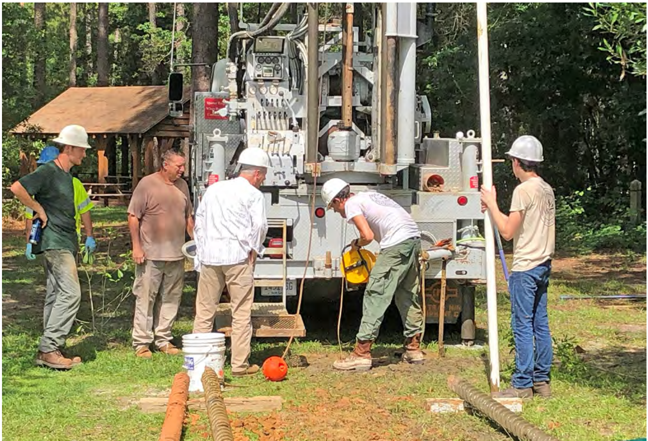
Figure 30. The South Carolina Geological Survey assisted in drilling a water-table well (COL-0803) at Colleton State Park in Colleton County.
