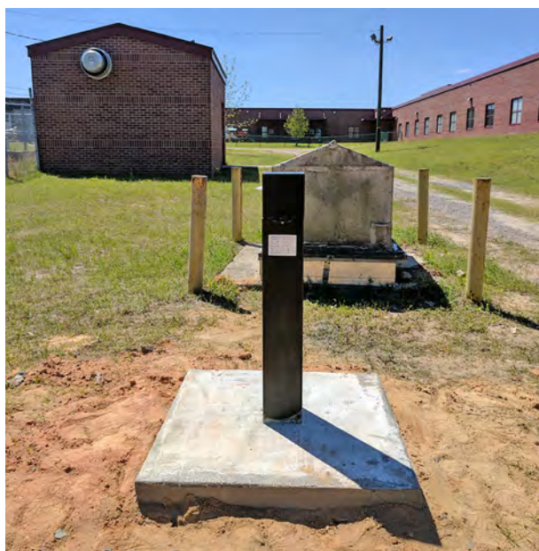
Figure 21. New monitoring well AIK-2733 at Oakwood-Windsor Elementary School in Aiken County. The well is screened in the Gordon aquifer (170 ft deep).
