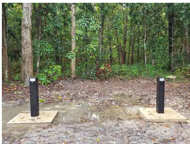
Figure 19. New monitoring wells at Myrtle Beach State Park in Horry County. HOR-1326 (left) is screened in the McQueen Branch aquifer (600 feet deep) and HOR-1327 (right) is screened in the Crouch Branch aquifer (440 feet deep). HOR-1327 is also part of the Saltwater Intrusion Monitoring Network.
