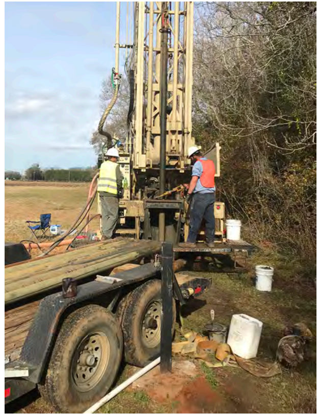
Figure 27. Drilling the new deep well (CAL-0215) at the Creston cluster site.
