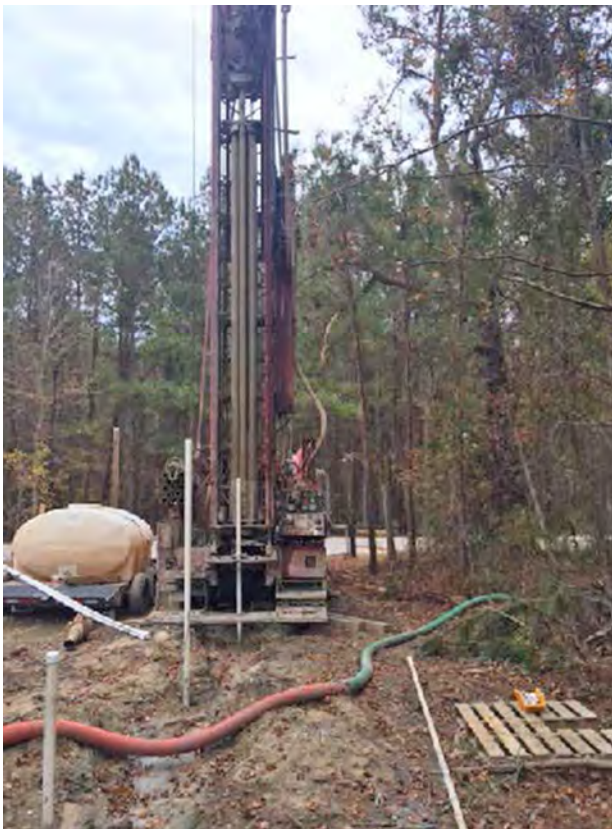
Figure 22. Installation of the 2" PVC well casings at the Sumter cluster site.
