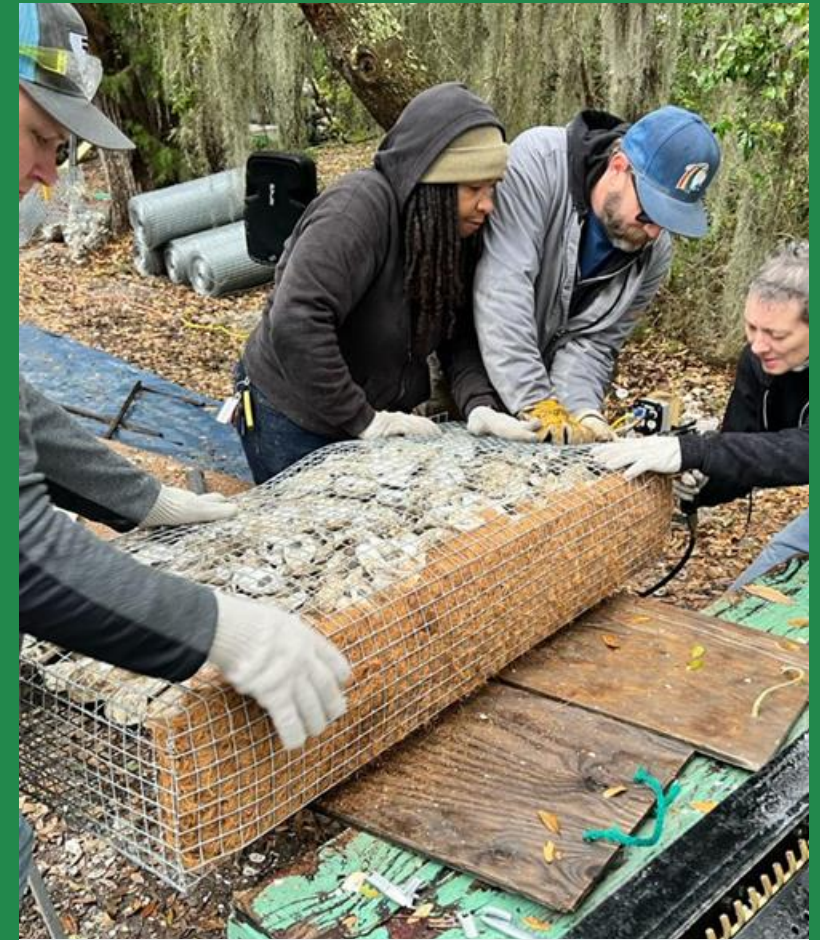
SCDNR volunteers make a Modified Wire Reef (MWR) - Photo Credit SCDNR
