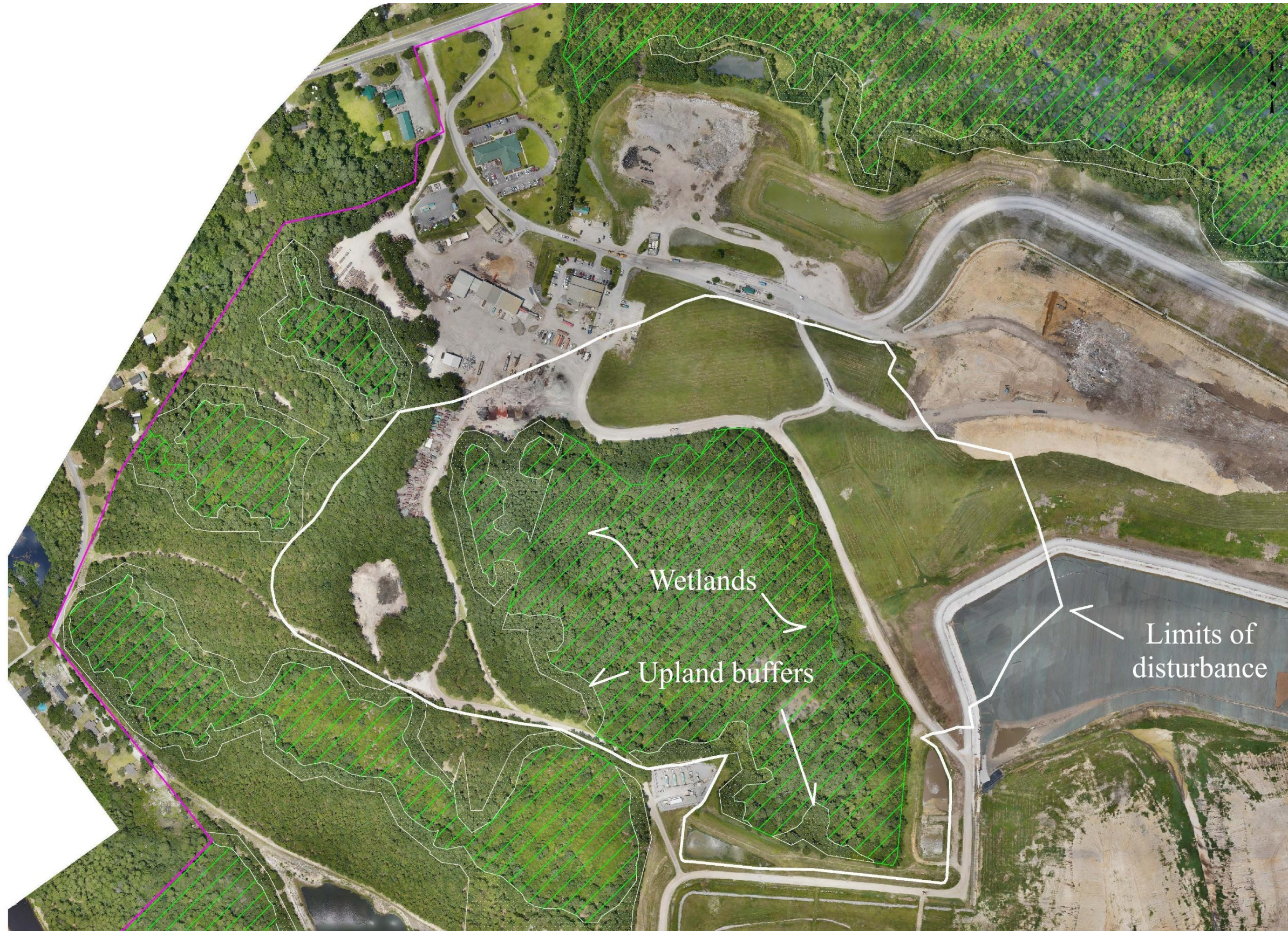
Figure 7. Aerial photograph showing the location of C&D Site 1. This 85-acre area contains 30.7 acres of wetlands and 4.85 acres of upland buffers, all of which are protected under restrictive covenants.
