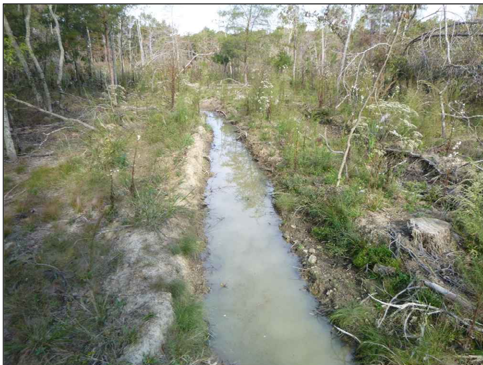
Figure 2.8. Water on surface within the deep tire ruts related to logging activities, facing northwest.
