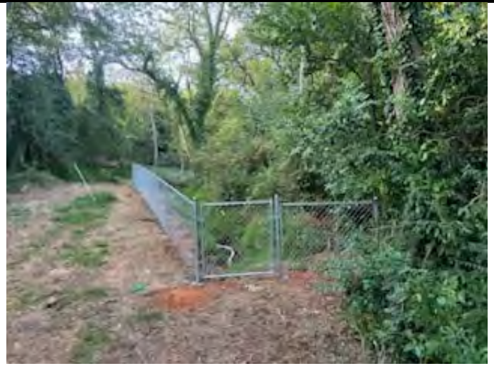
Trench Containment Fence
