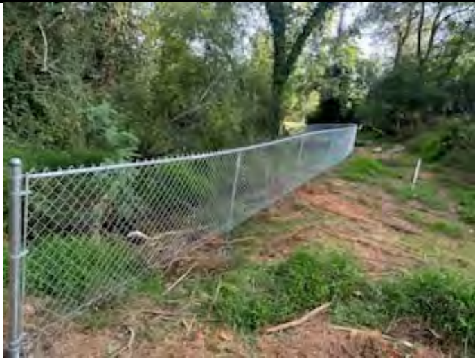
Trench Containment Fence
