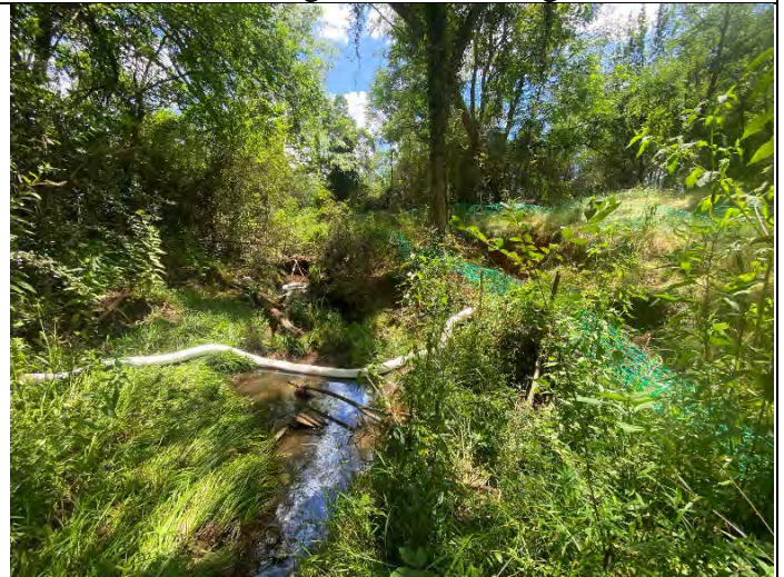
New Boom #1 Installed Across Drainage Creek
