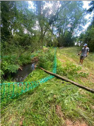
Old Boom Removal
