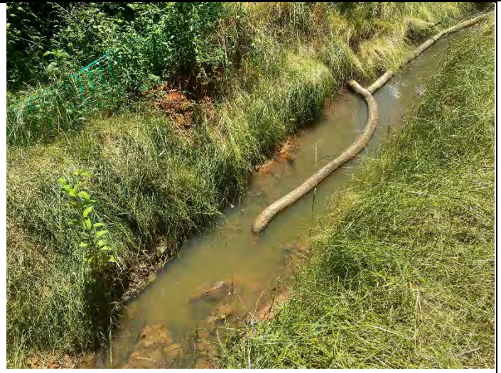
Southern Excavation Area Old Booms
