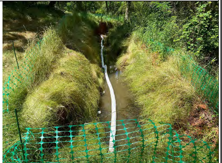
New Boom Installed in Southern Excavation Looking North.
