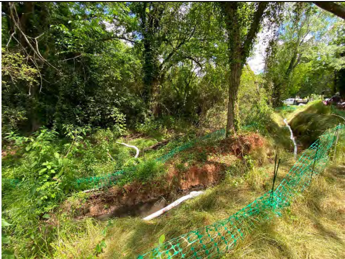
New Booms Installed.
