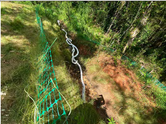
Additional Booms Installed Northern Excavation.
