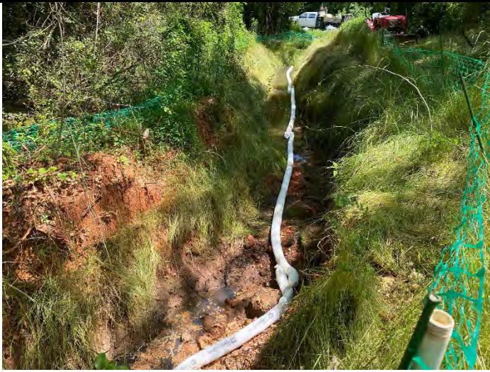
New Boom Installed Southern Excavation.
