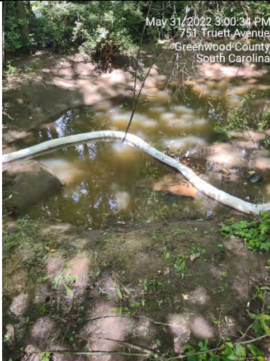
New Boom #4 Installed in Pond.
