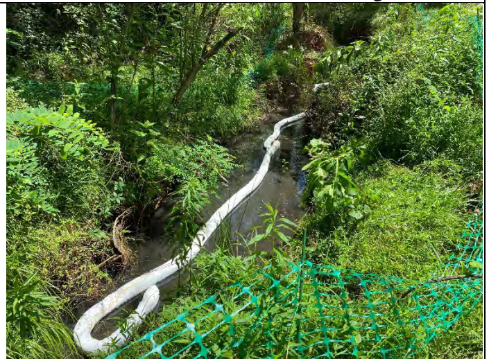
New Boom Installed in Northern Excavation Original Pit Location.
