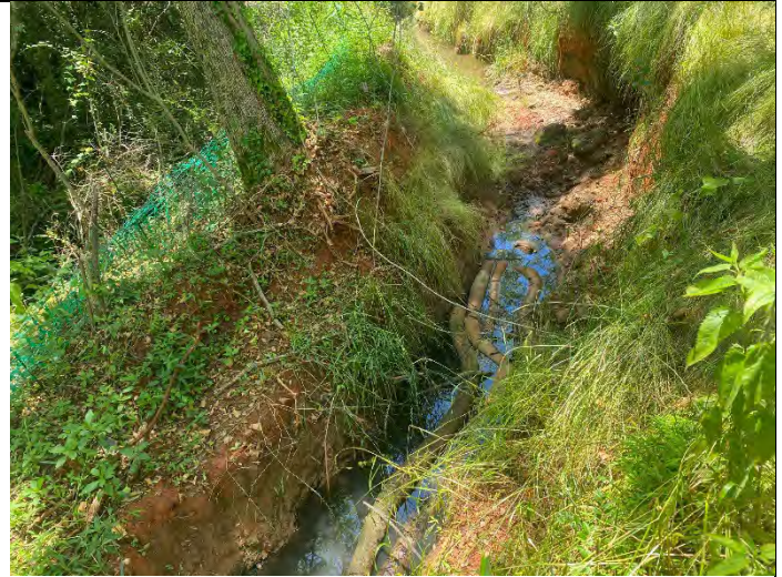
Northern Excavation Area Old Booms
