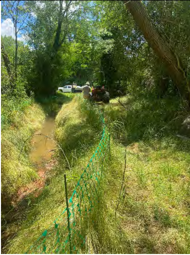
Old Booms Removed Southern Excavation.
