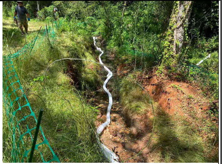
New Boom Installed Northern Excavation.
