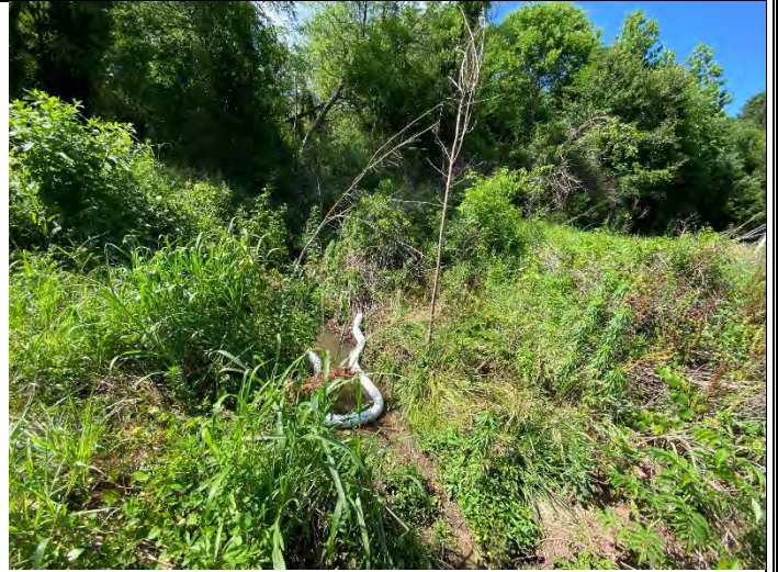
New Boom #3 Installed in Drainage Creek.
