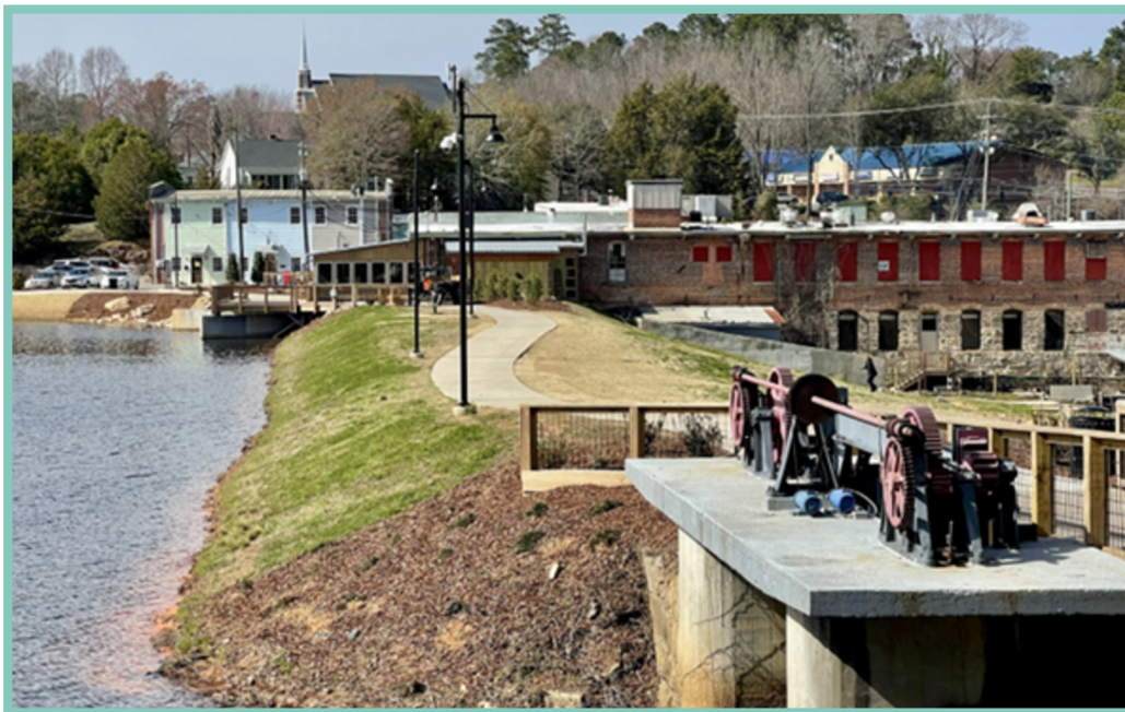
The Lexington Old Mill Pond Dam, one of the dams to breach during the historic 2015 flood event, held a ribbon cutting ceremony to celebrate the official opening of the 1.15-mile trail that now encircles the pond in September 2024.
