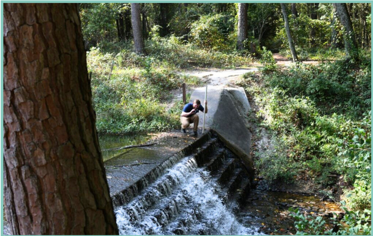
An SCDES dam inspector assesses a High Hazard dam built by the Civilian Conservation Corps in the 1930s.
