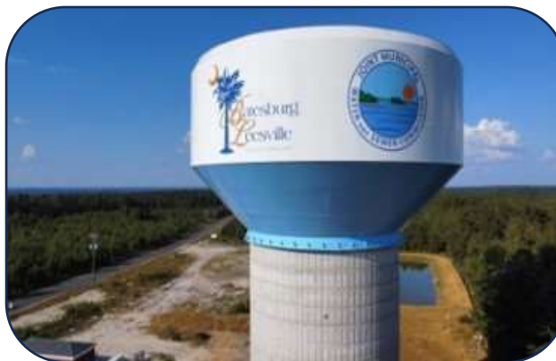
Elevated water tank built through a partnership between JMWSC and the Town of Batesburg-Leesville. (Photo provided by RIA.)
