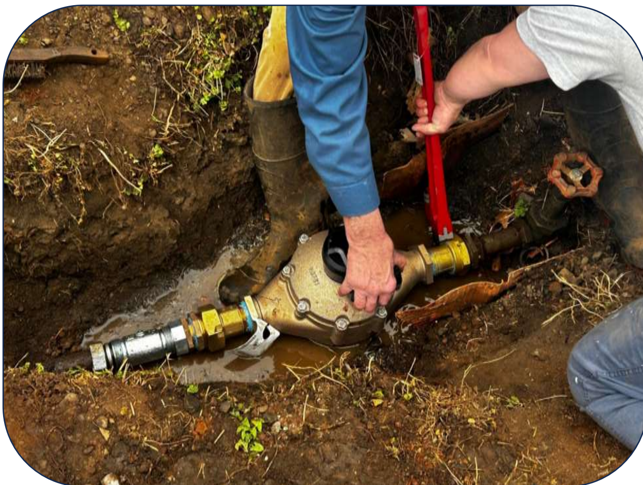
SCRWA staff assist the Town of Lockhart by teaching the proper technique for large water meter replacement. (Photo provided by SCRWA, April 2026)
