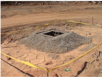
Block and Gravel Inlet Protection
