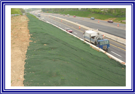
TRM Slope Application
