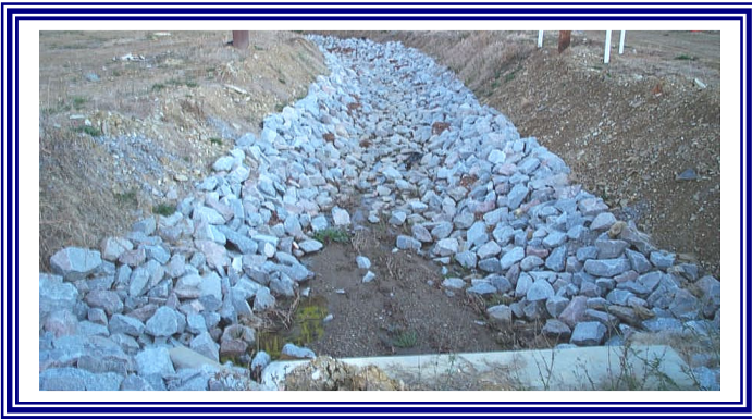
Riprap Lined Channel
