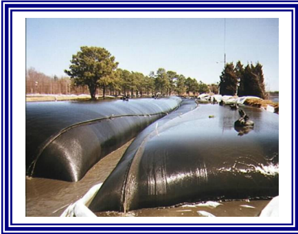
Construction Dewatering
