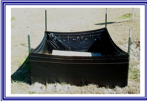
Filter Fabric Inlet Protection
