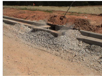
Block and Gravel Inlet Protection
