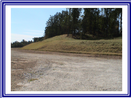
Temporary Slope Stabilization
