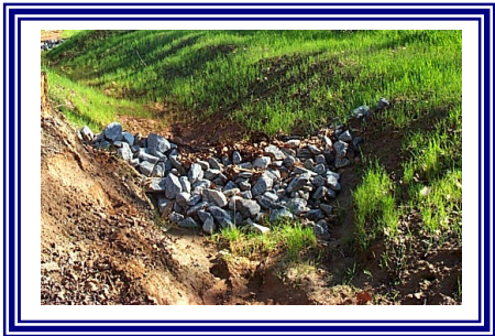
Rock Check Dam
