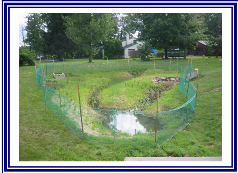
Established Storm Water Wetland
