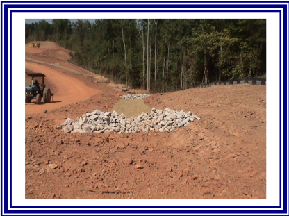
Rock Check Dam
