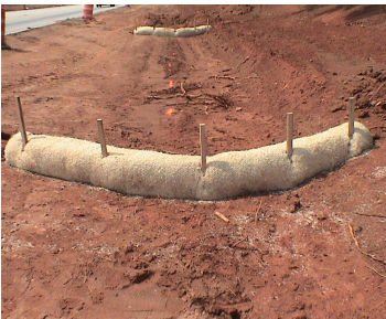
Sediment Tube Check Dam
