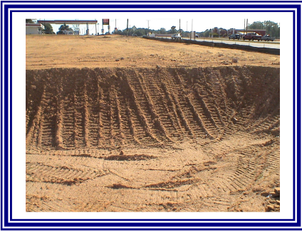
Surface Roughening (Tracking)
