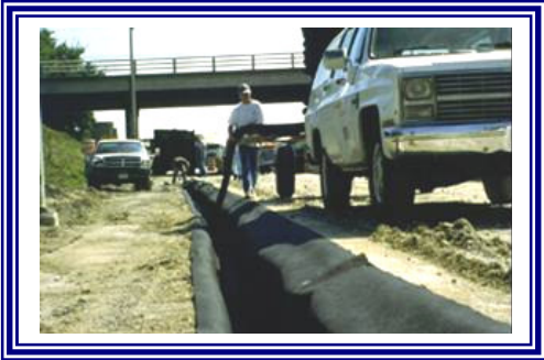
Subsurface Drain
