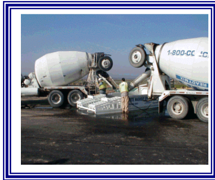
Concrete Truck Washout
