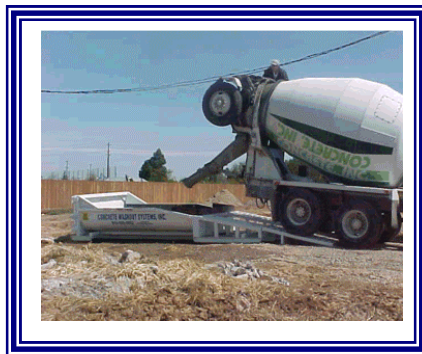
Concrete Truck Washout
