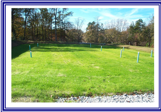
Bioretention Area with un-cut clean outs
