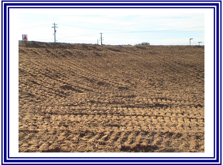
Surface Roughening (Tracking)
