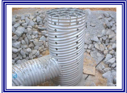
Sediment Basin Perforated Riser
