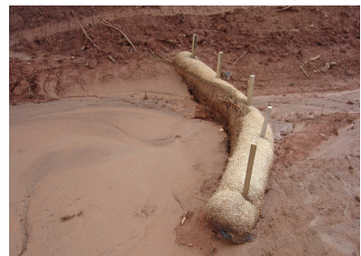
Sediment Tube Check Dam
