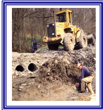
Temporary Stream Crossing
