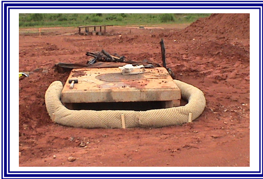
Sediment Tube Inlet Protection
