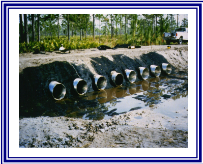
Temporary Stream Crossing
