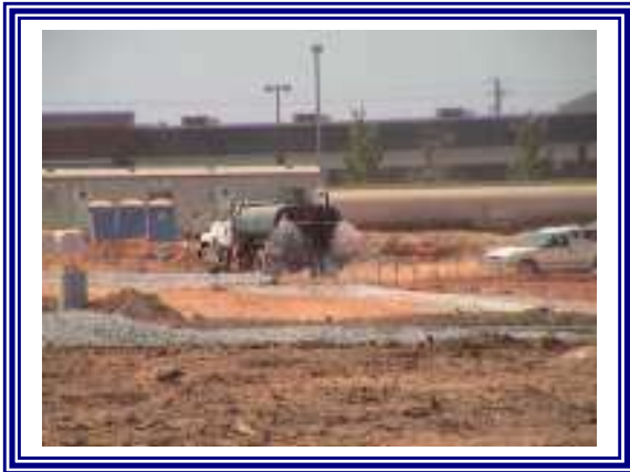
Dust Control by Sprinkling Water
