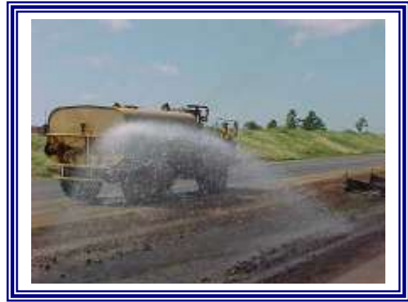
Dust Control by Sprinkling Water
