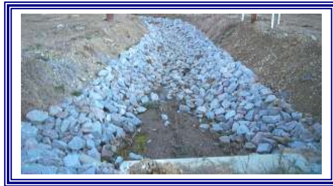
Riprap Lined Channel
