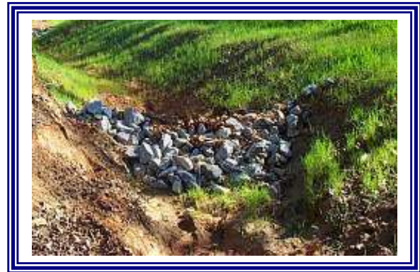
Rock Check Dam
