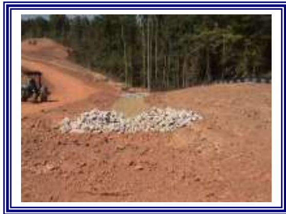
Rock Check Dam
