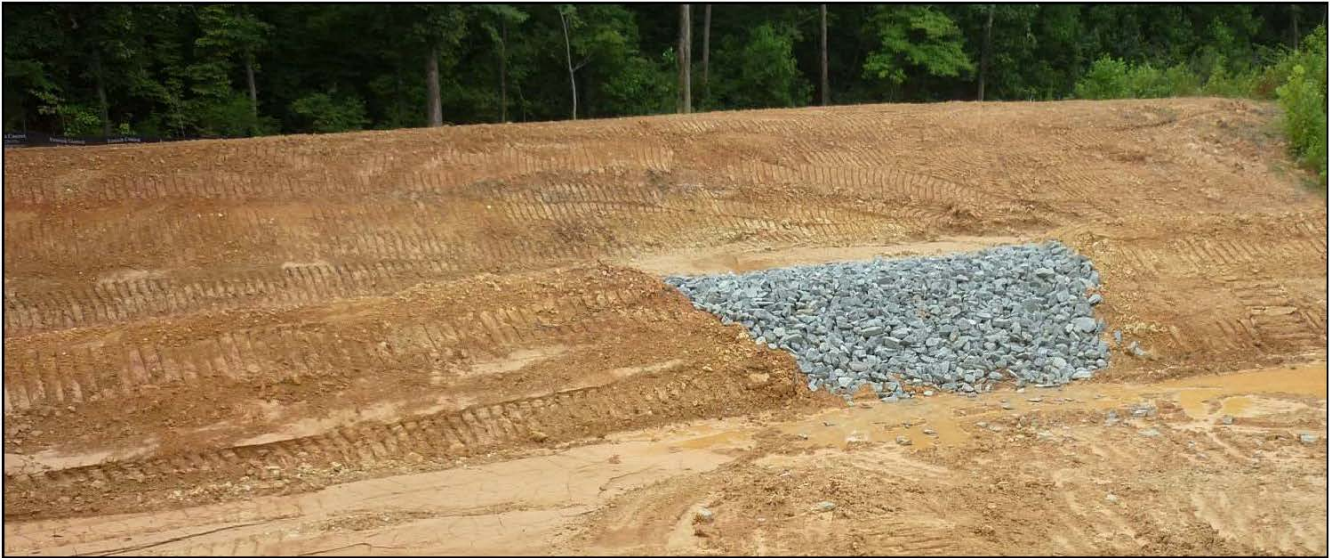
Photo: Sediment Forebay
