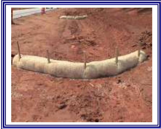
Sediment Tube Check Dam
