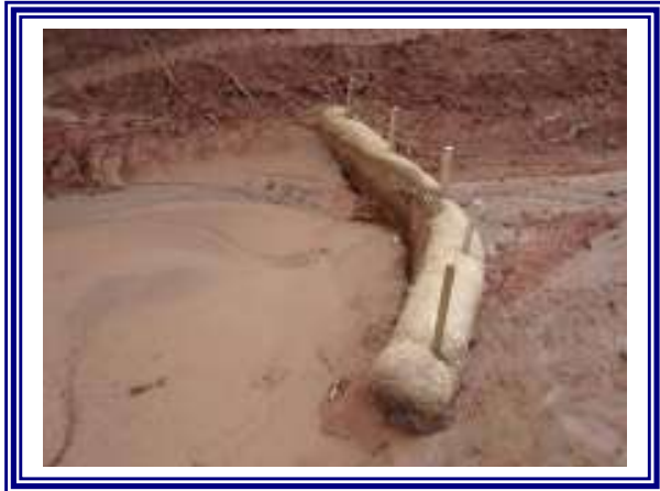
Sediment Tube Check Dam
