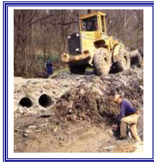
Temporary Stream Crossing
