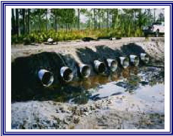
Temporary Stream Crossing
