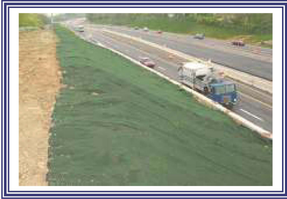
TRM Slope Application
