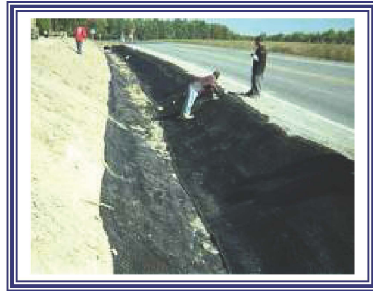
TRM Channel Application
