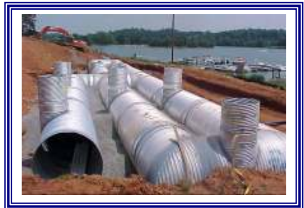
CMP Underground Detention
