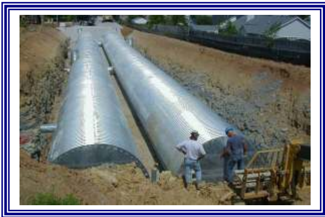
CMP Underground Detention
