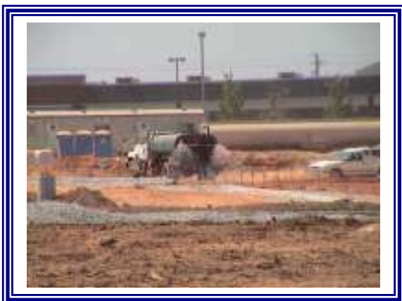
Dust Control by Sprinkling Water
