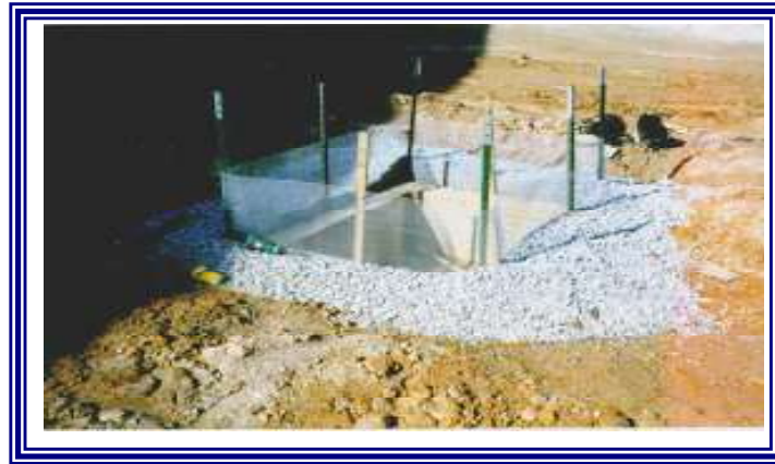
Hardware Fabric and Stone Inlet Protection
