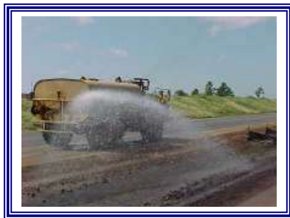
Dust Control by Sprinkling Water
