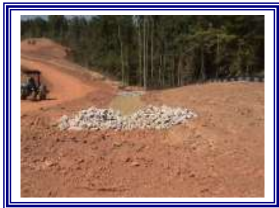
Rock Check Dam
