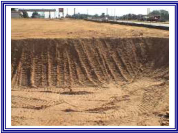
Surface Roughening (Tracking)
