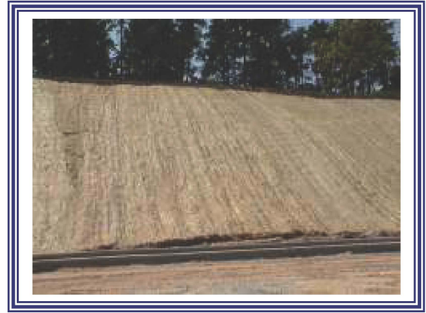
ECB Slope Application
