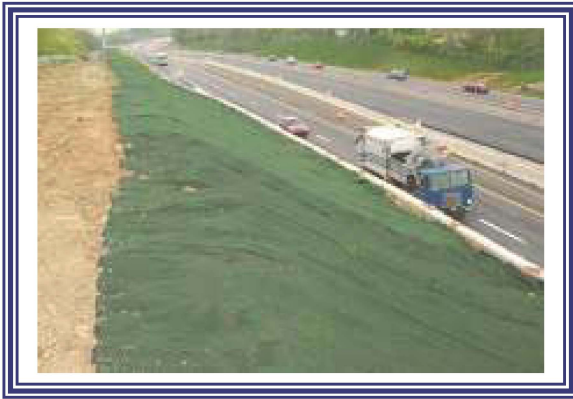
TRM Slope Application
