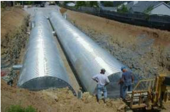
CMP Underground Detention
