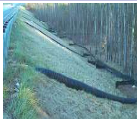
Pipe Slope Drain
