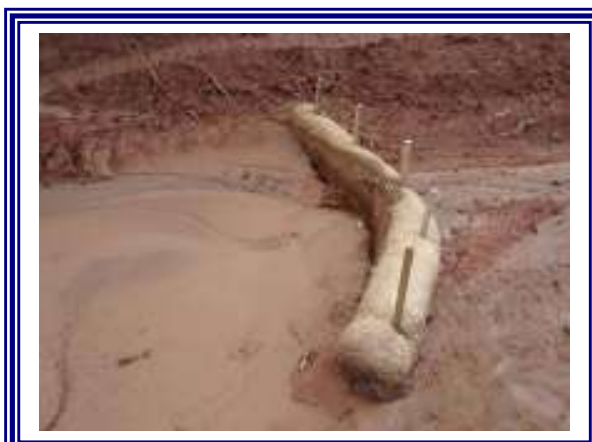
Sediment Tube Check Dam
