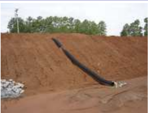
Pipe Slope Drain
