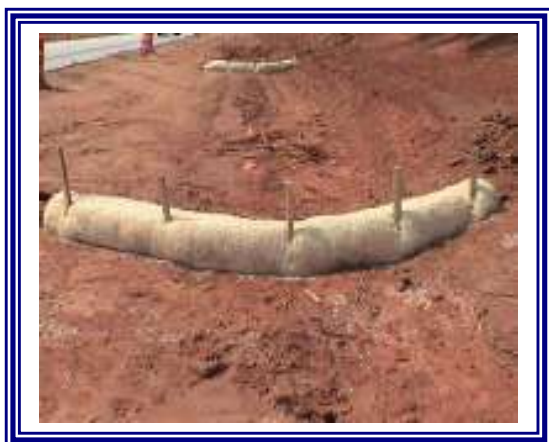
Sediment Tube Check Dam
