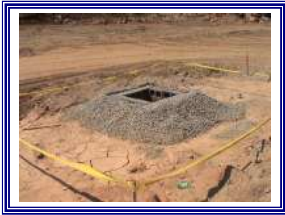
Block and Gravel Inlet Protection
