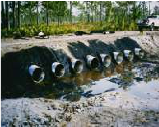
Temporary Stream Crossing
