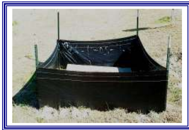
Filter Fabric Inlet Protection
