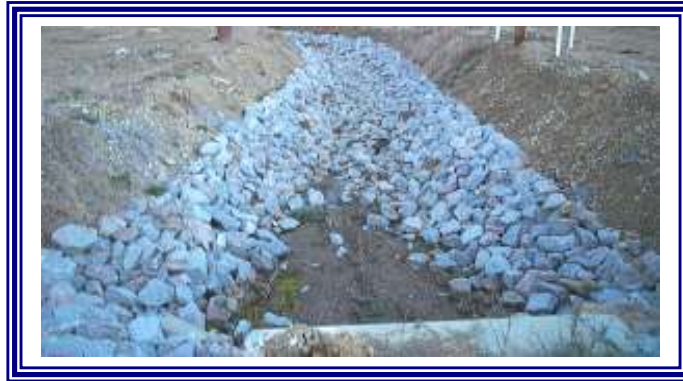
Riprap Lined Channel
