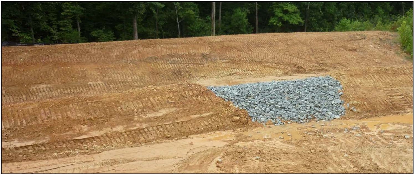
Photo: Sediment Forebay
