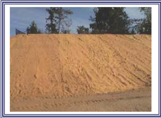
ECB Slope Application
