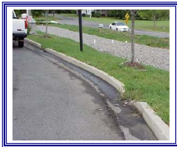
Infiltration Trench
