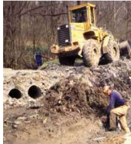
Temporary Stream Crossing
