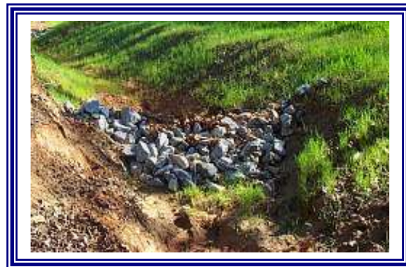
Rock Check Dam
