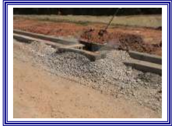
Block and Gravel Inlet Protection
