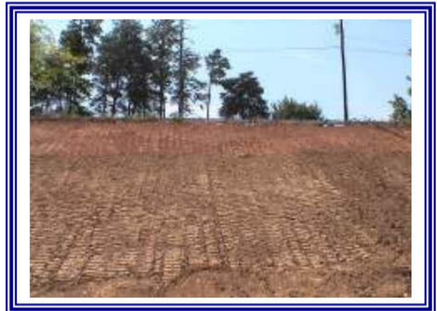
Surface Roughening (Tracking)
