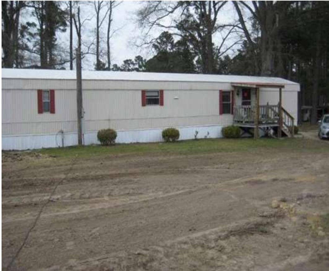
Figure 5. The same property after septic repair
