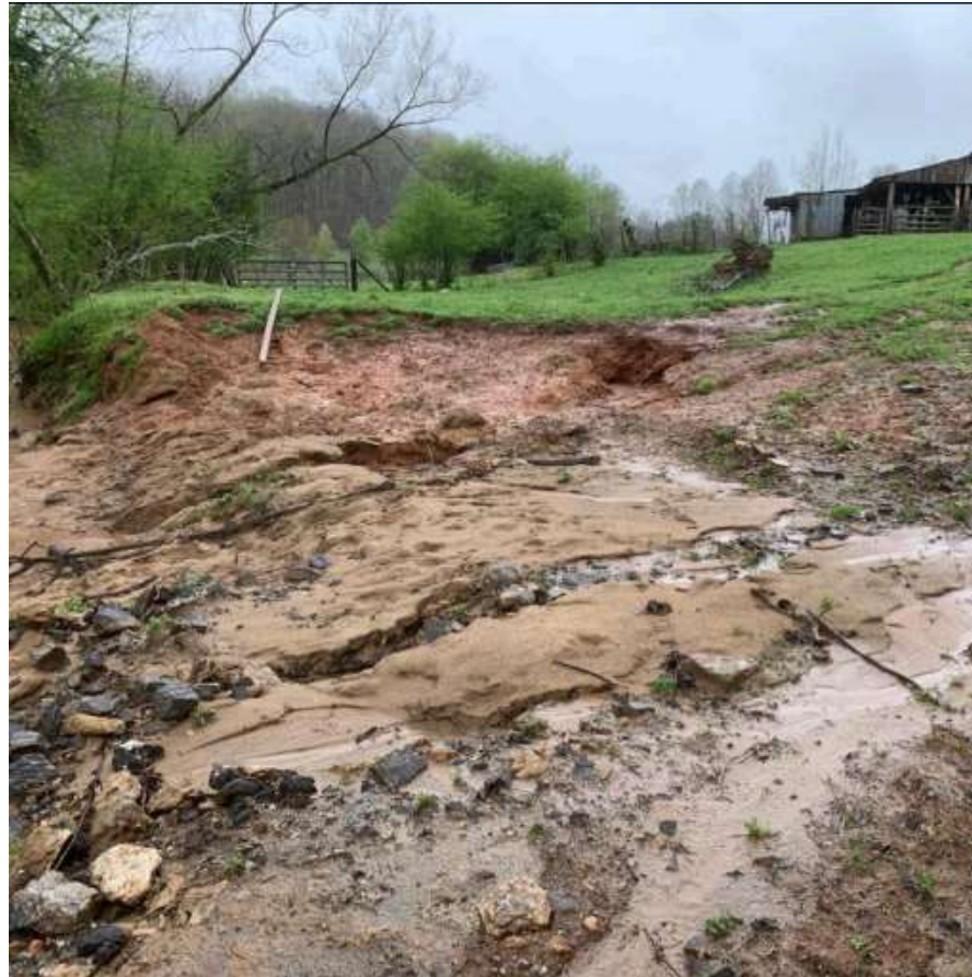
Figure 3. Erosion eliminated streambank buffers
