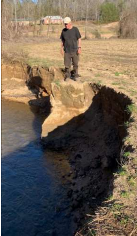
Figure 4. Significant channel erosion
