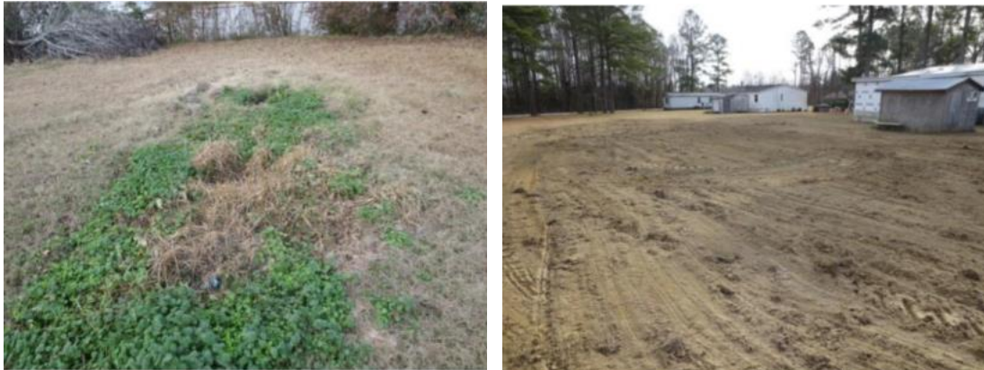
Before and after the repair of a failing septic system
