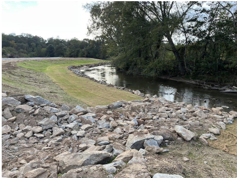
Rock-lined waterway constructed with donated blast rock
