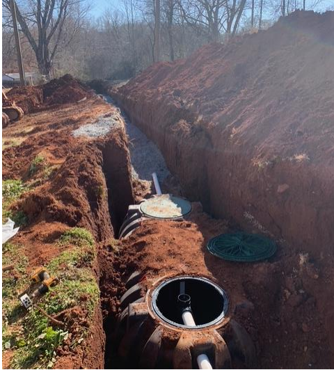
Septic tank replacement
