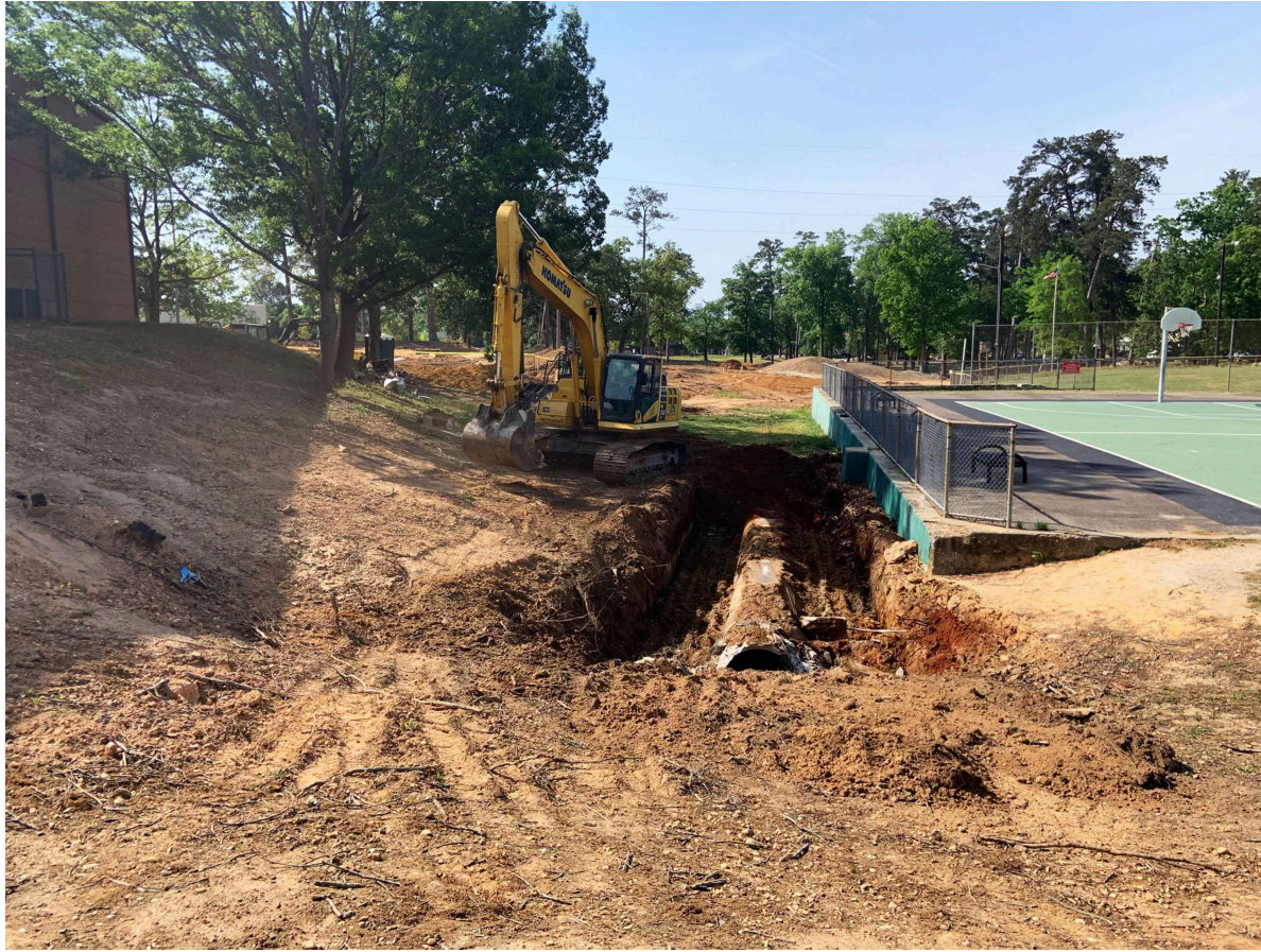
Figure 4. Excavation of the piped Smith Branch tributary
