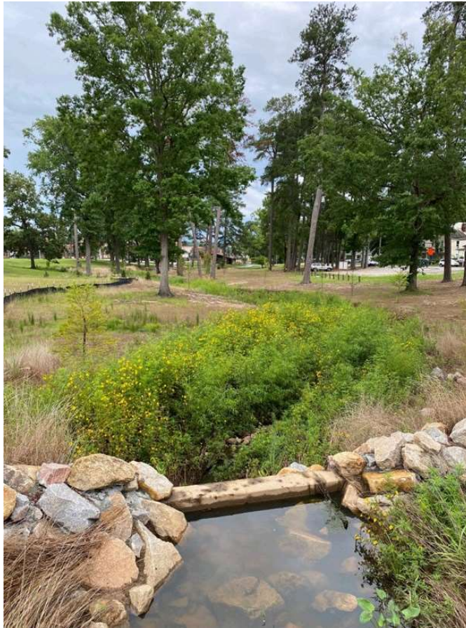
Figure 5. Daylighted stream in Hyatt Park after construction.
