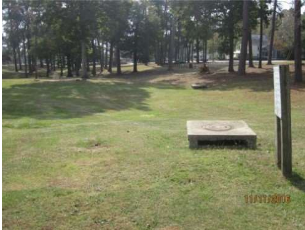
Figure 3. Path of storm drains in Hyatt Park before stream daylighting.
