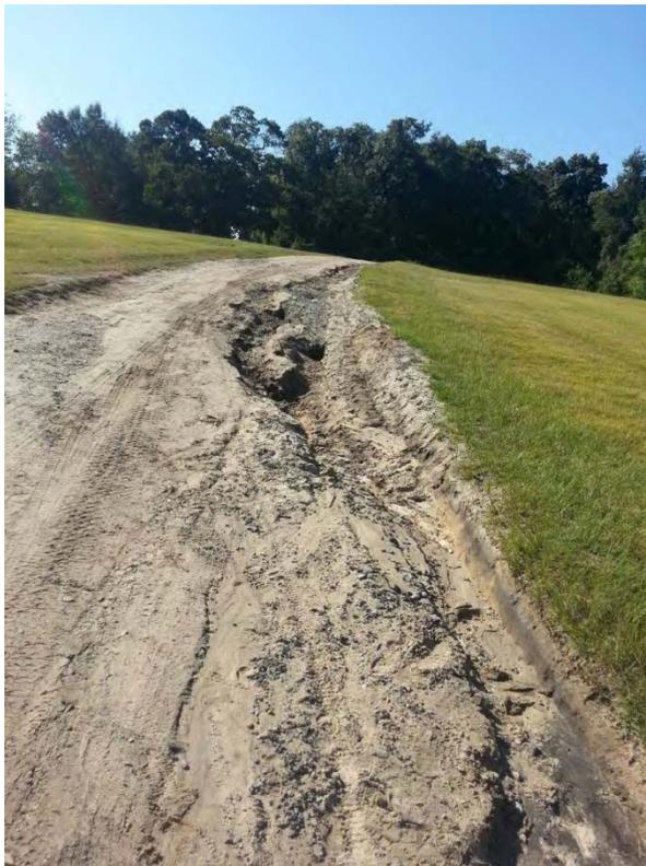
**Figure 8. Erosion on Gravel Road at Children’s Garden at Clemson Extension**
