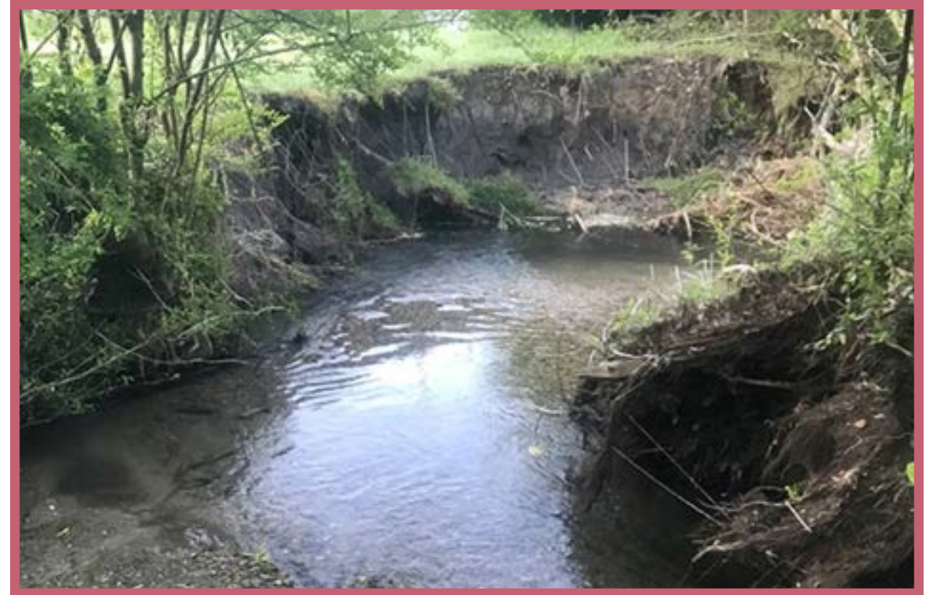
Figure 2.14 Streambank erosion caused by hydrologic impacts (Clemson University)
