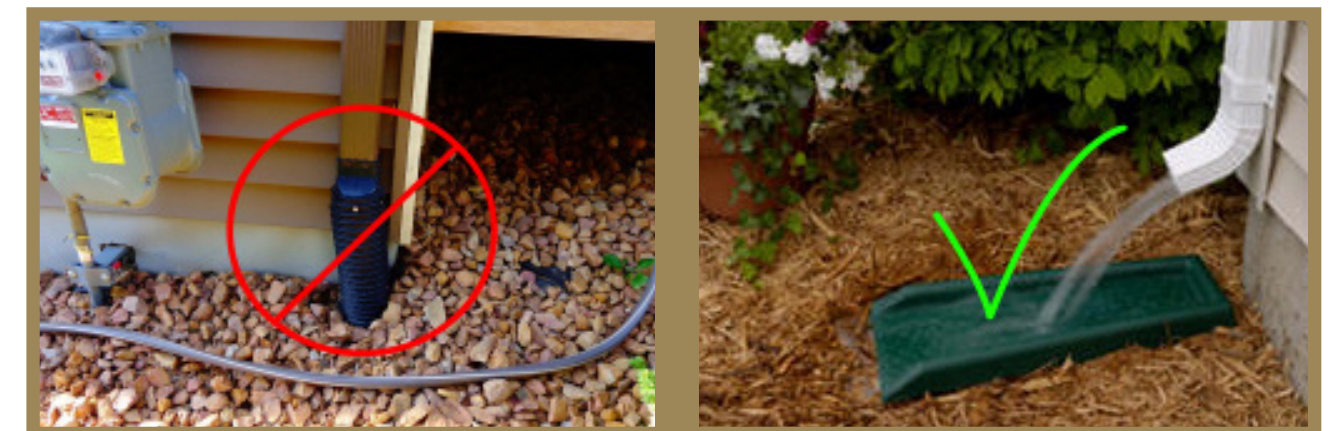
Figure 5.27 Downspout disconnect allows stormwater to recharge groundwater (The Pocket)
