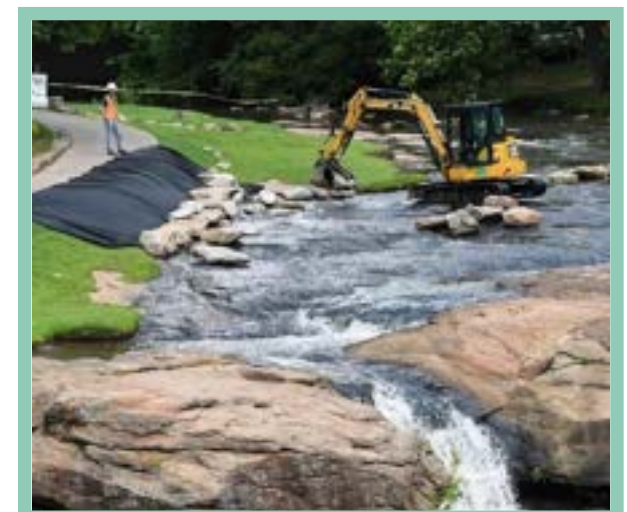
Figure 6.9 Stream restoration in Falls Park, SC (Greenville News)
