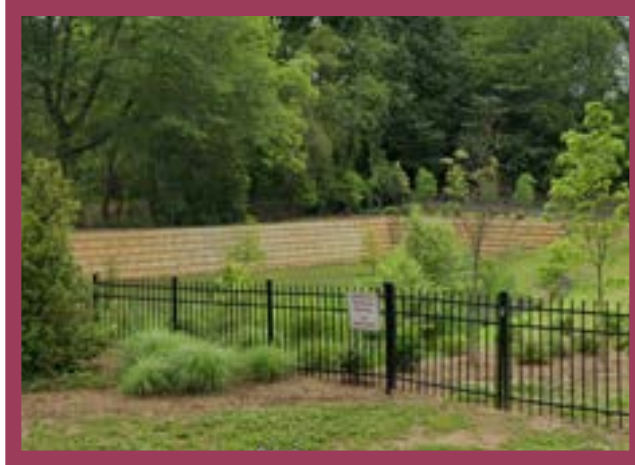
Figure 1.27 Completed Detention Basin on College Ave (City of Rock Hill)
