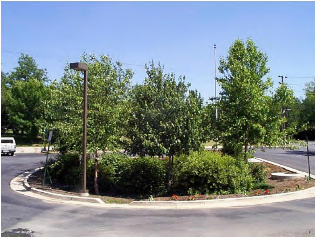
Figure 4-8. Bioretention in a Parking Lot Turnaround
