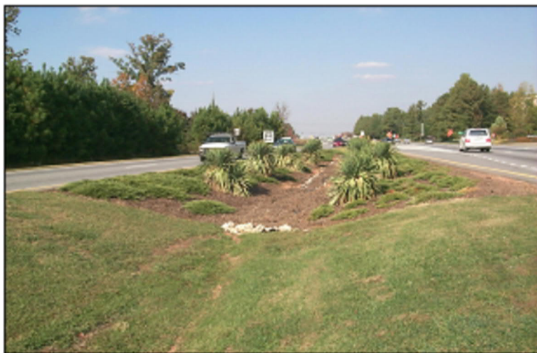
Figure 4-20. Enhanced Dry Swale
