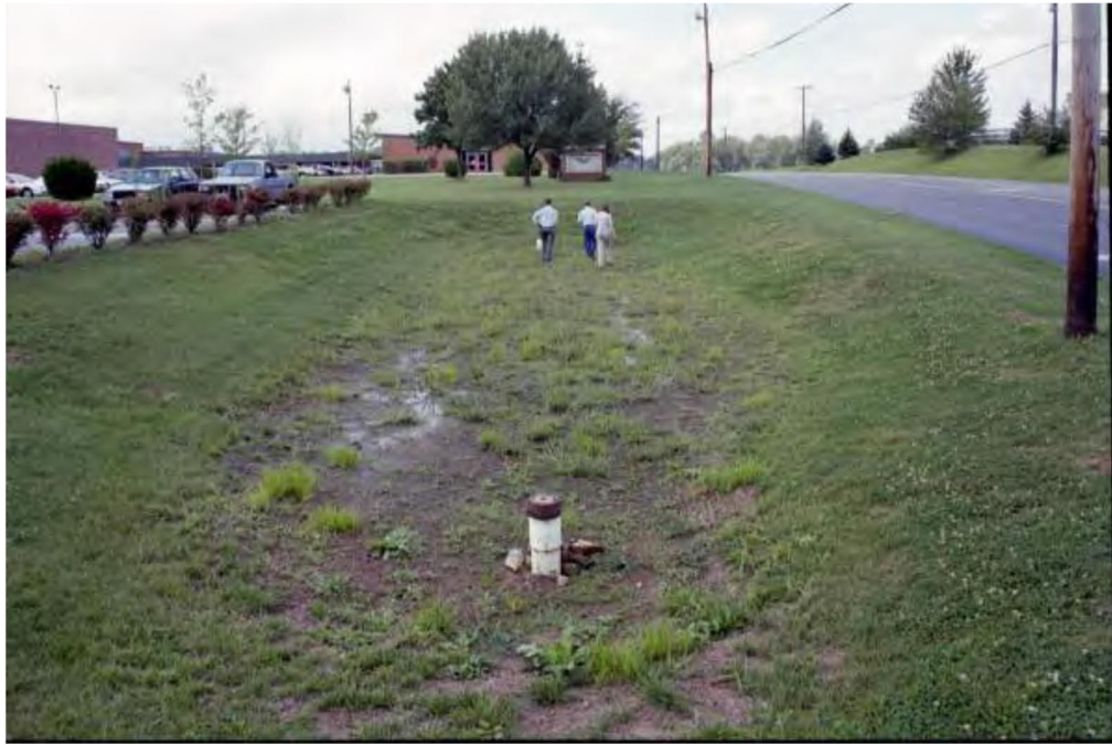
Figure 4-12. Surface Sand Filter
