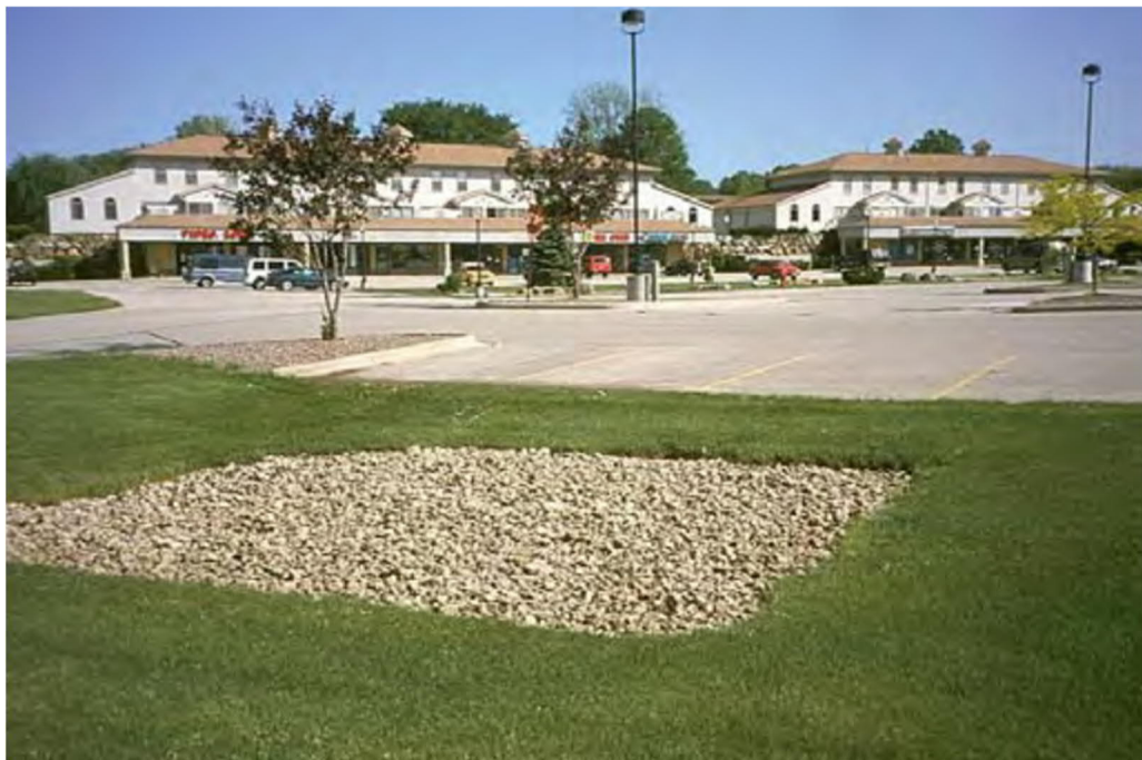
Figure 4-17. Grass Filter Pretreatment for an Infiltration Trench
