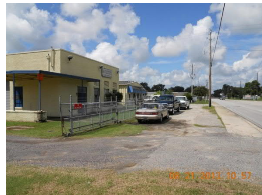
Figure 3-3. Darlington Street Water Plant
