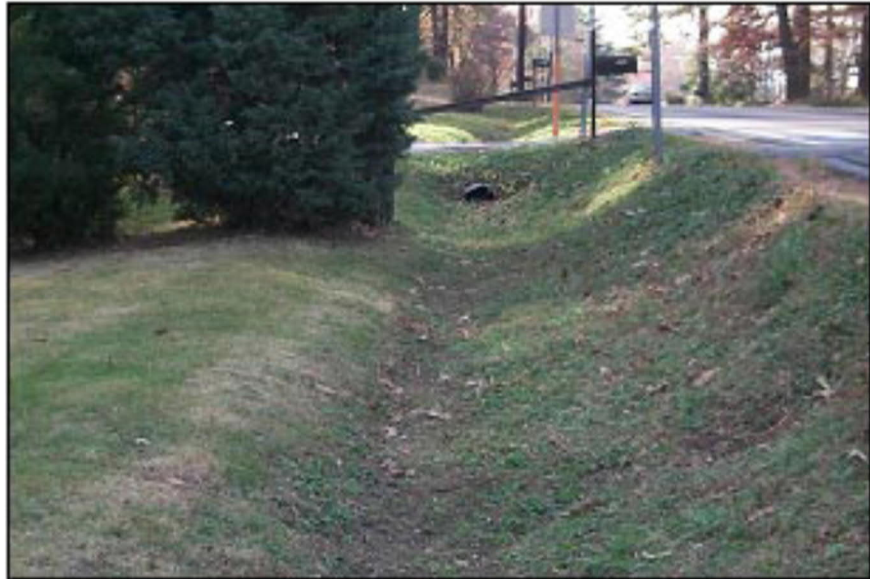
Figure 4-15. Grass-Lined Open Channel
