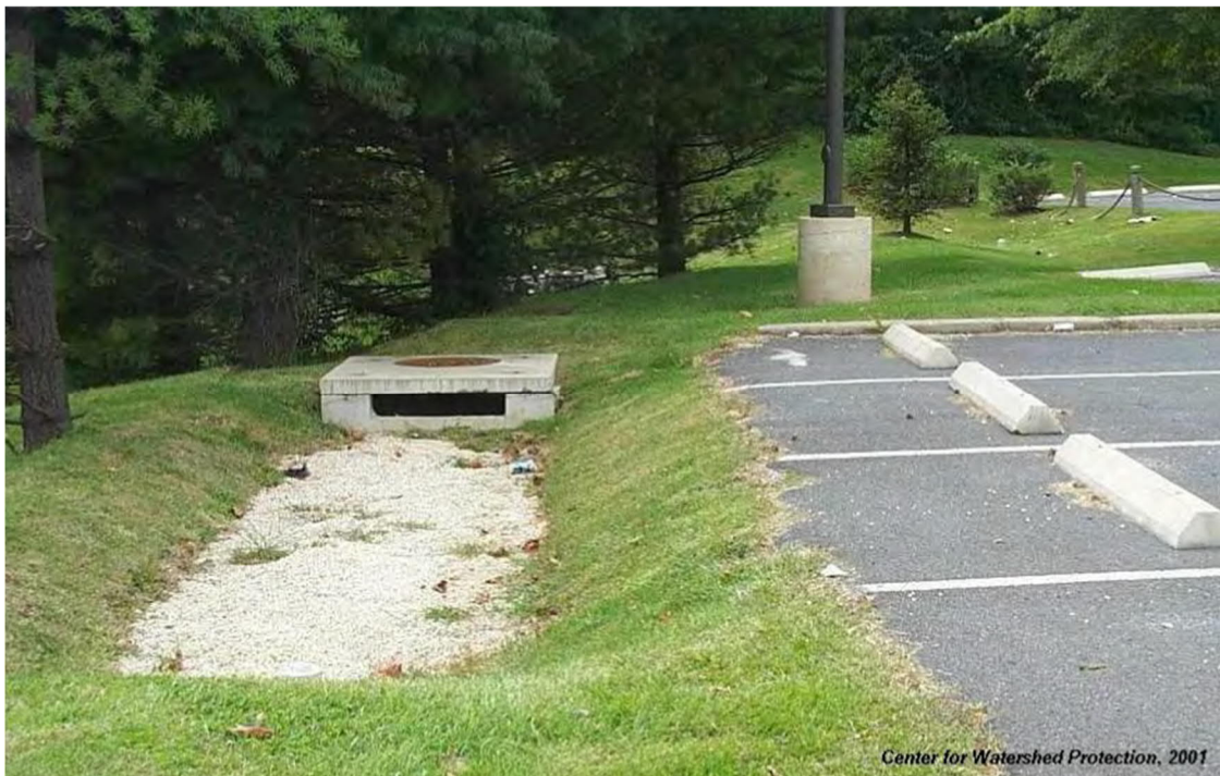
Figure 4-10. Infiltration Trench
