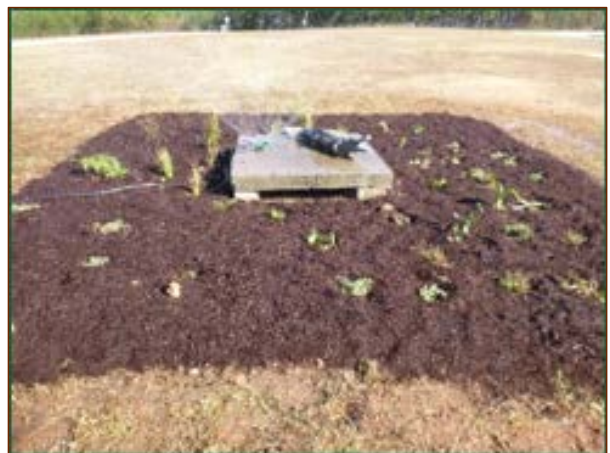
Examples of pervious pavement and rain garden installed around stormwater inlet
