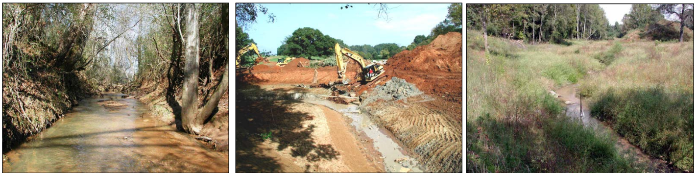
Example of a Riparian Buffer Restoration in Hunnicutt Creek, Clemson University – Channelized Stream Overrun With Invasive Species,, During Construction, After Restoration (Source: Clemson University)
