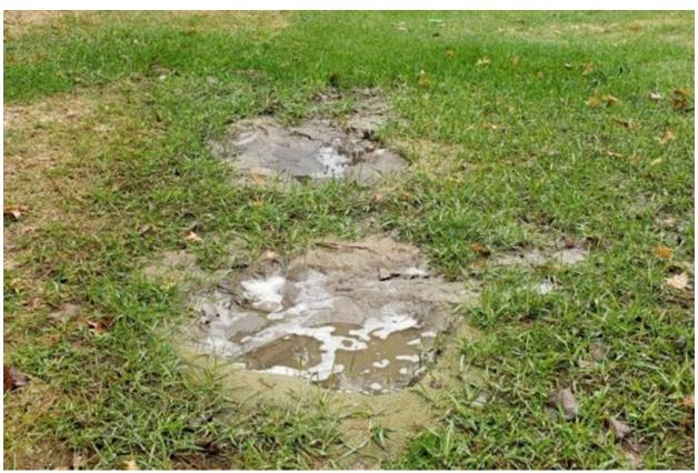
Photo 8: Example of Failing Septic System (photo credit: Wexco Environmental)
