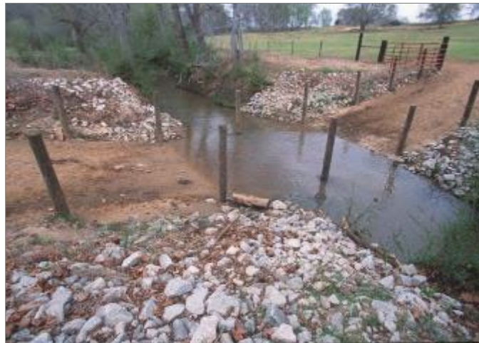
Armored Streambank Crossing.
