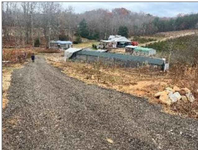
Example of farm road stabilization in the Tyger River Watershed.
