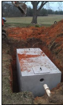
Example of Septic Tank Replacement
