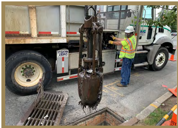
Figure 5.8 Cleaning dirty catch basins in the Big Apple (NYC Environmental Protection)
