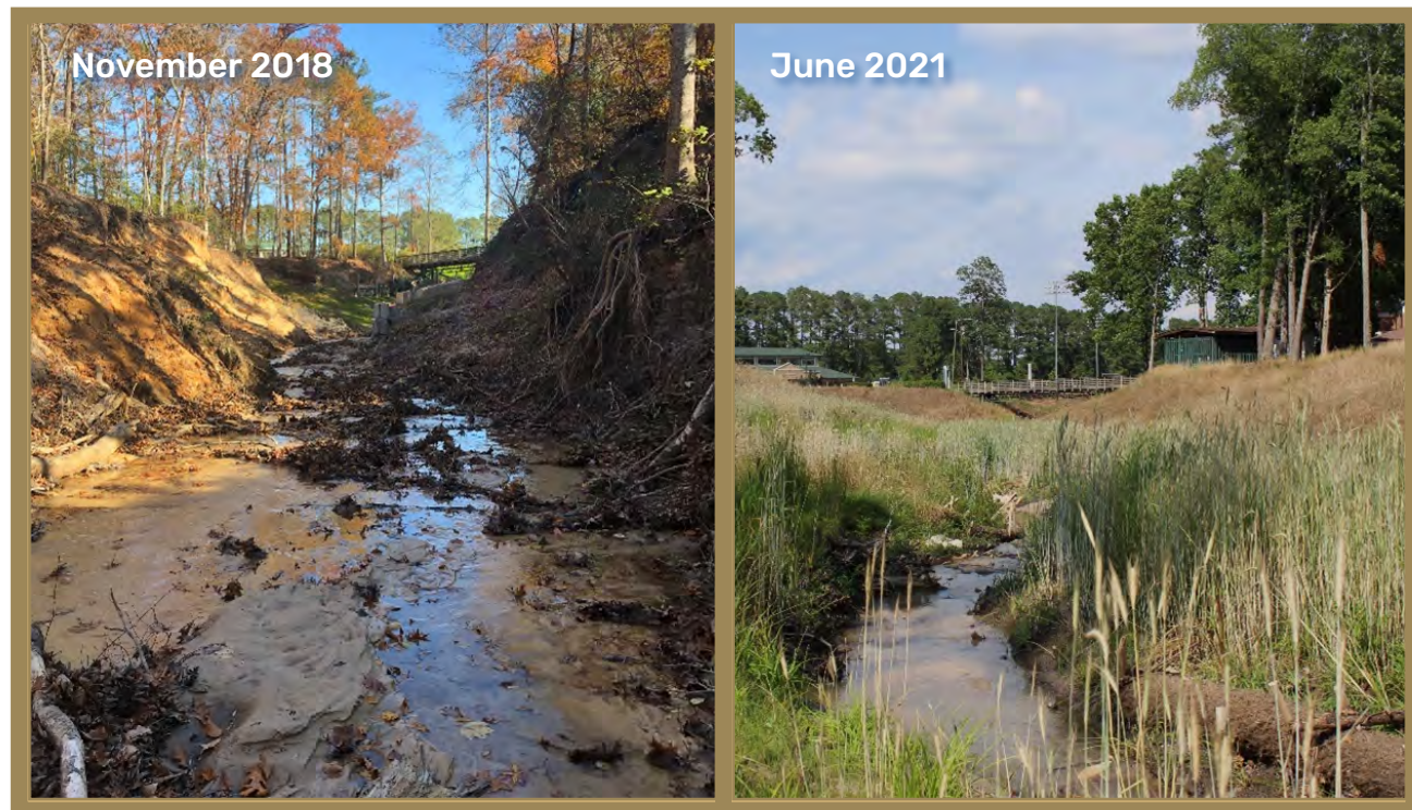
Figure 5.35 Before and after, Methodist University stream restoration (McAdams)
