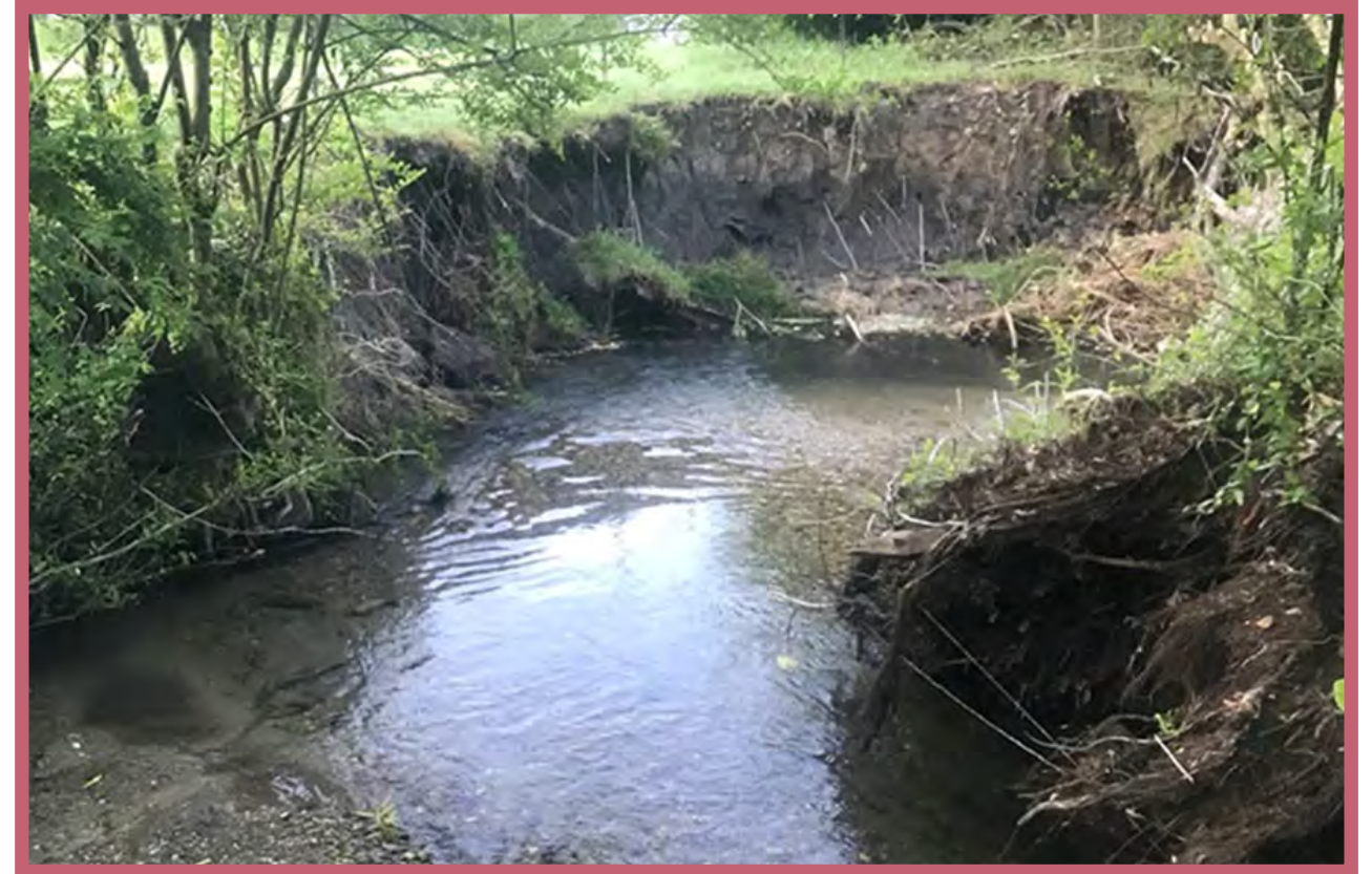
Figure 2.17 Streambank erosion caused by hydrologic impacts (Clemson University)
