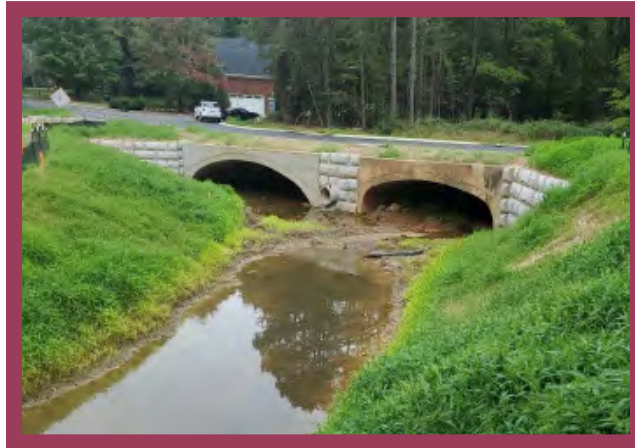
Figure 1.26 Completed Cavendale Dr. Stream Retoration (City of Rock Hill)
