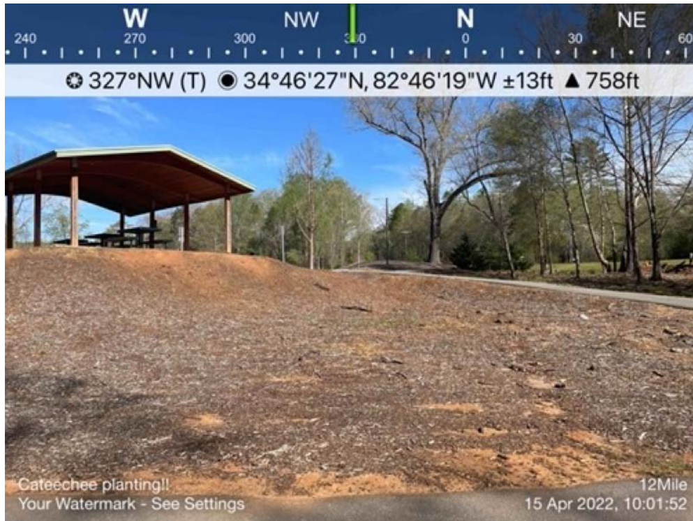
Fig. 46. The picnic shelter at Cateechee Point Park provides a great opportunity to demonstrate low impact landscaping design and ecological improvements that would also better manage the ongoing soil erosion.
