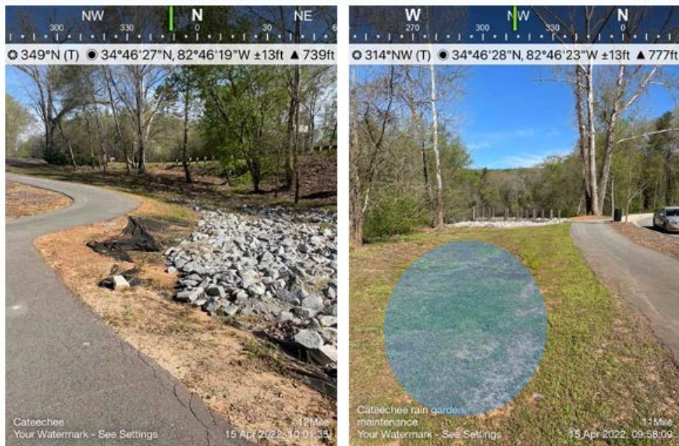
Fig. 45. Two rain garden opportunities for improved stormwater pollution prevention and enhanced groundwater storage. The right most image includes an area depicting the observed low point for stormwater capture and treatment.
