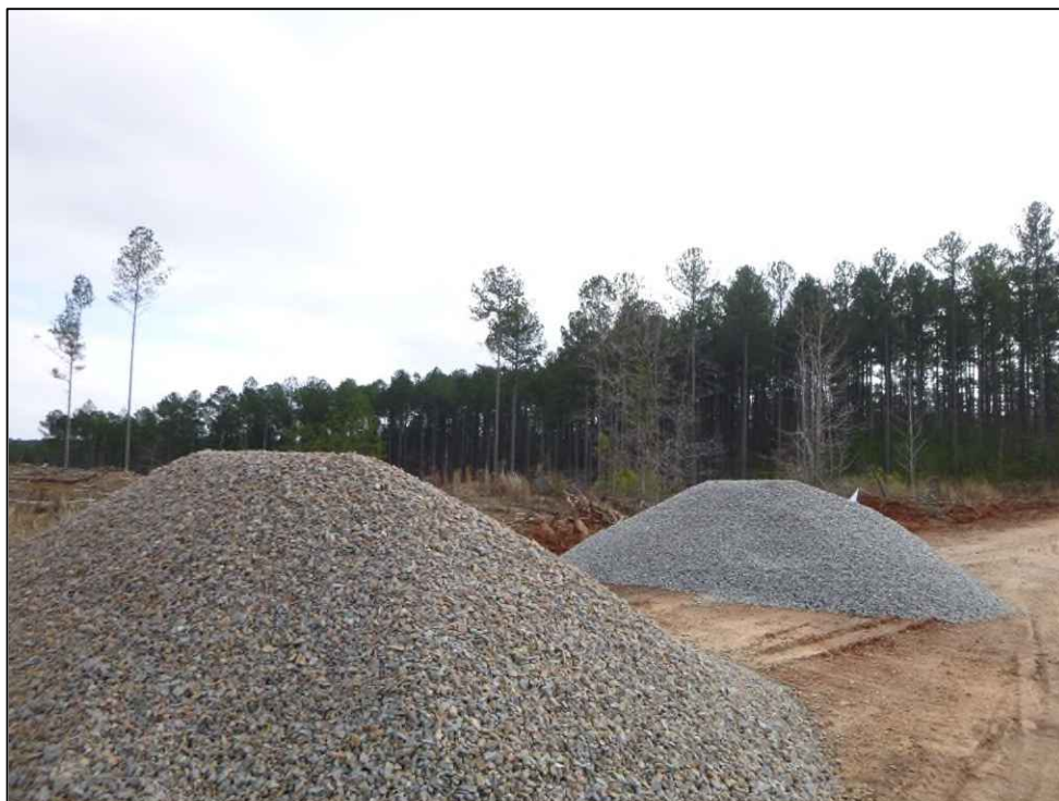
Figure 2.8. Gravel piles within the project area, facing southeast.
