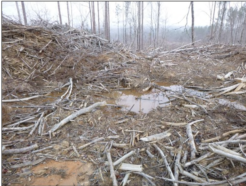
Figure 2.7. Typical push pile/timber pile within the project area, facing northwest.
