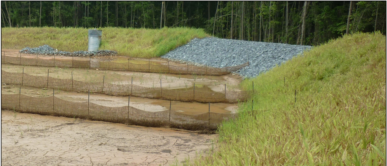
Photo: Porous Baffles
