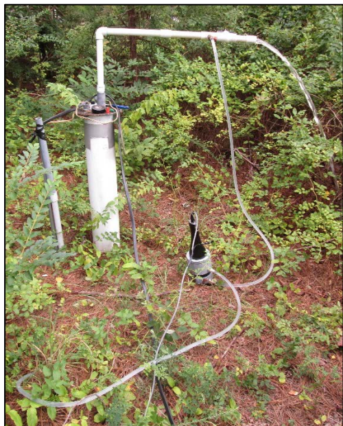
Above: Cluster well being pumped and tested for water perimeters
