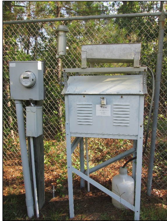
Example of an Air Monitoring Station with Rain Collection Pans and Glass Fiber Filters (on top) and Silica Gel Columns (inside)
