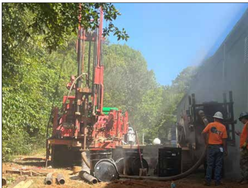
A groundwater monitoring well being installed at the Columbus Industries Site in FY24.
