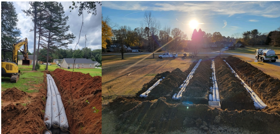
Fig. 35. Examples of septic repair work in the Three and Twenty Creek watershed, which neighbors the Twelvemile River watershed. (photo provided by Upstate Forever).
