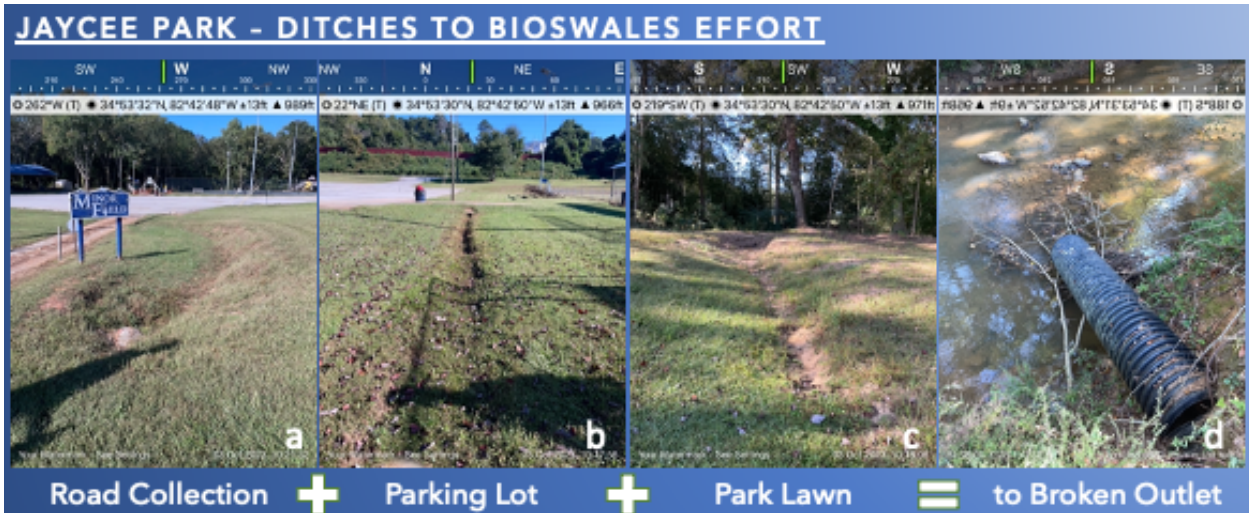
Fig. 43. Treatment train solution to stormwater runoff collection, ultimately reducing stormwater pollution in Town Creek.
