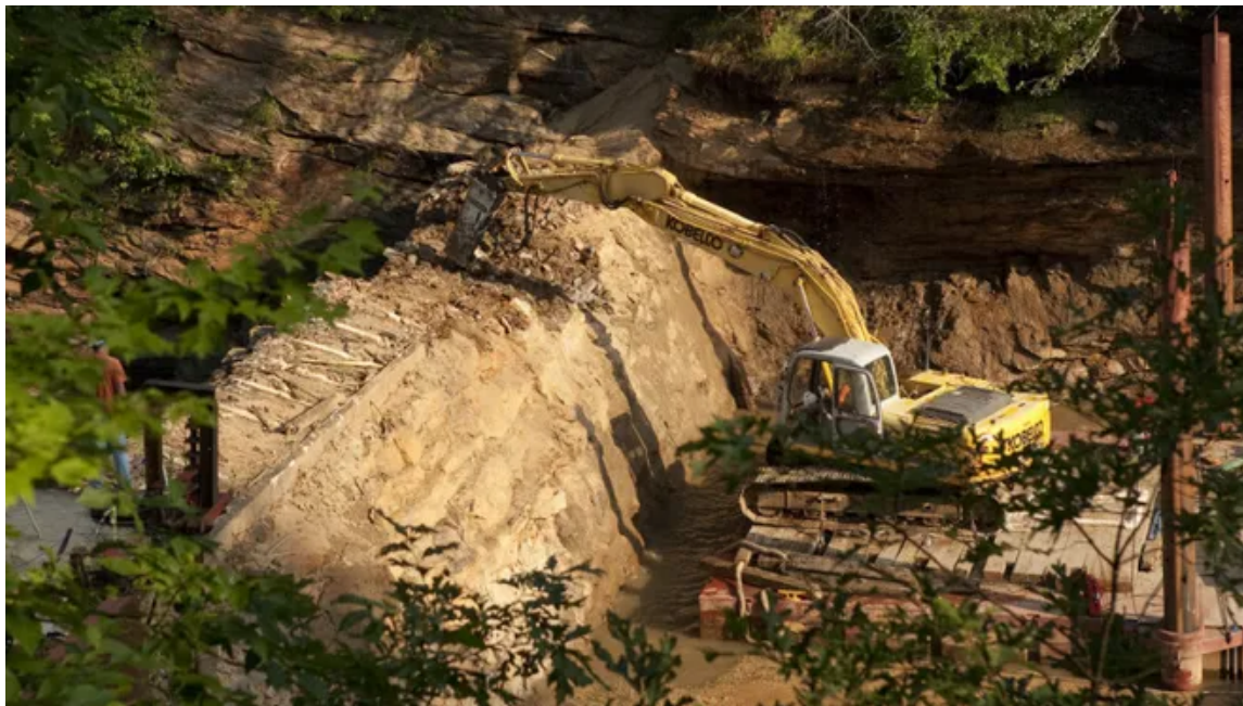
Fig. 8. Demolition of the Woodside II Dam in July 2011 (Photo: Greenville News)
