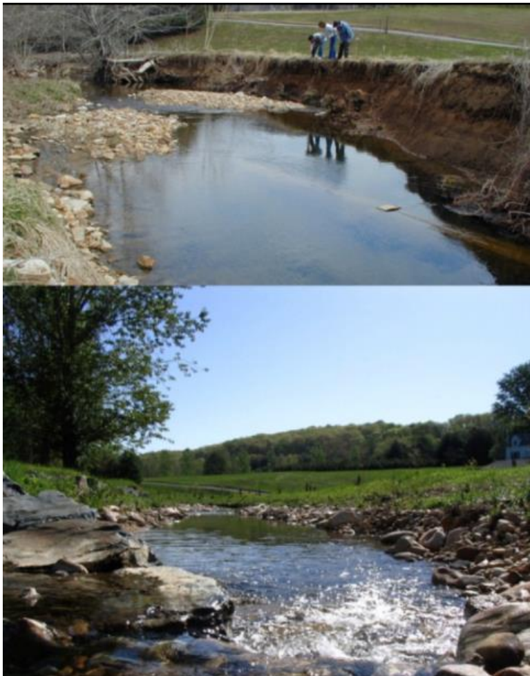
FIGURE 42: BEFORE AND AFTER PHOTOS FROM A STREAM STABILIZATION PROJECT
