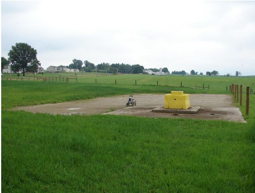
FIGURE 44 HEAVY USE AREA STABILIZATION PREVENTS OVERUSE OF LAND
