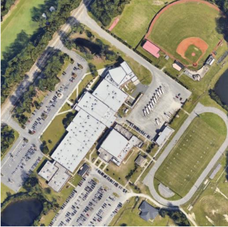
FIGURE 52: WACCAMAW HIGH SCHOOL HAS A VAST AMOUNT OF ROOFTOP AVAILABLE FOR RAINWATER HARVESTING
