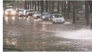
Repetitive Flooding on Victory Drive in Savannah, GA
