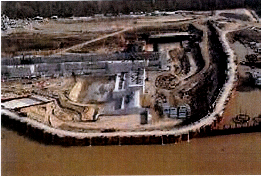
Figure 5 – Cofferd Dam Application
