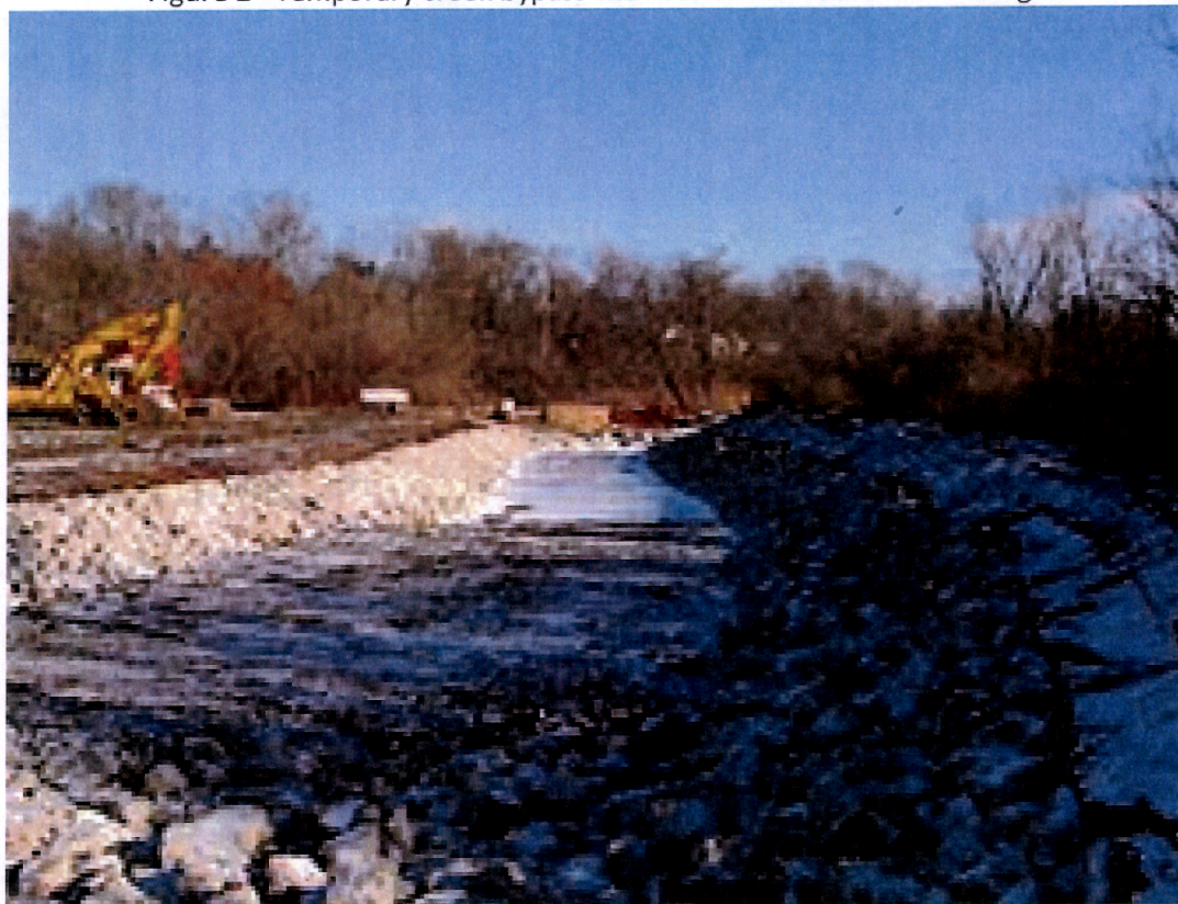
Figure 2 - Temporary creek bypass with Coffor Dam located to the right
