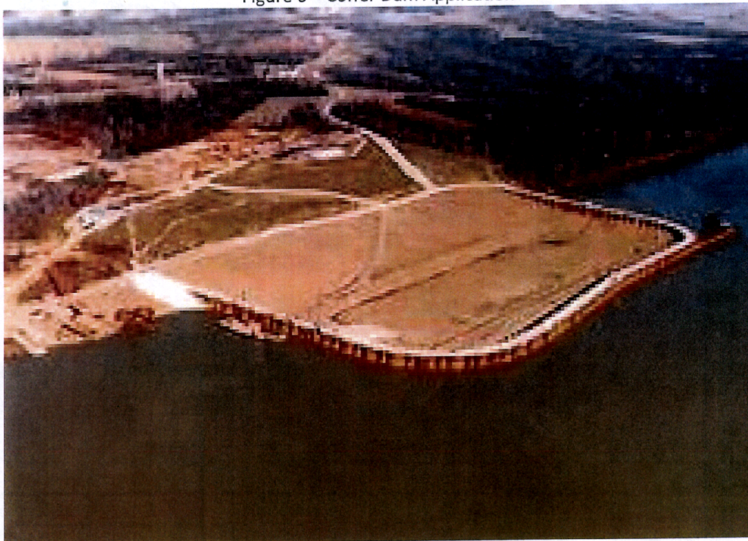
Figure 6 – Cofferd Dam Application
