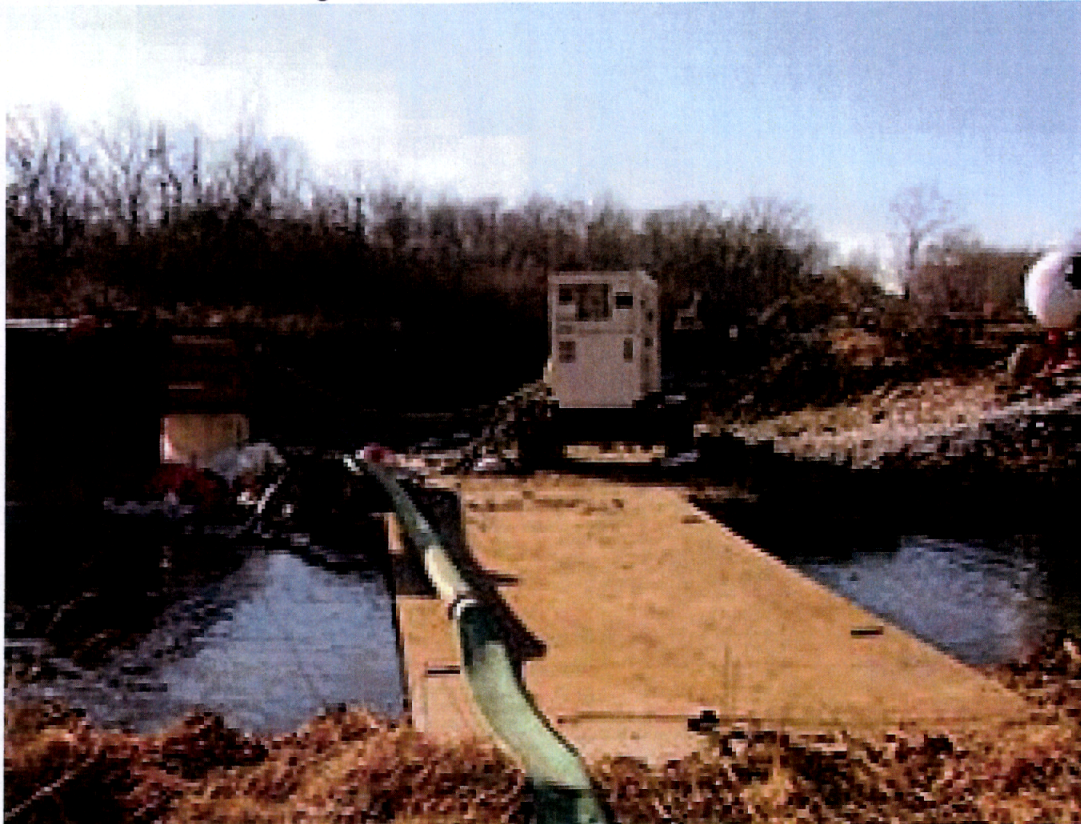
Figure 3 - Removal of stream bed sediment
