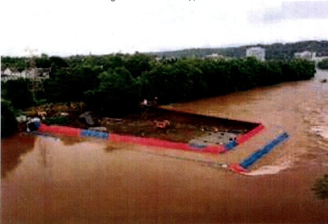
Figure 5 – Cofferd Dam Application
