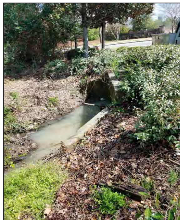
Outfall at SW-09 - West Side of Congaree River
