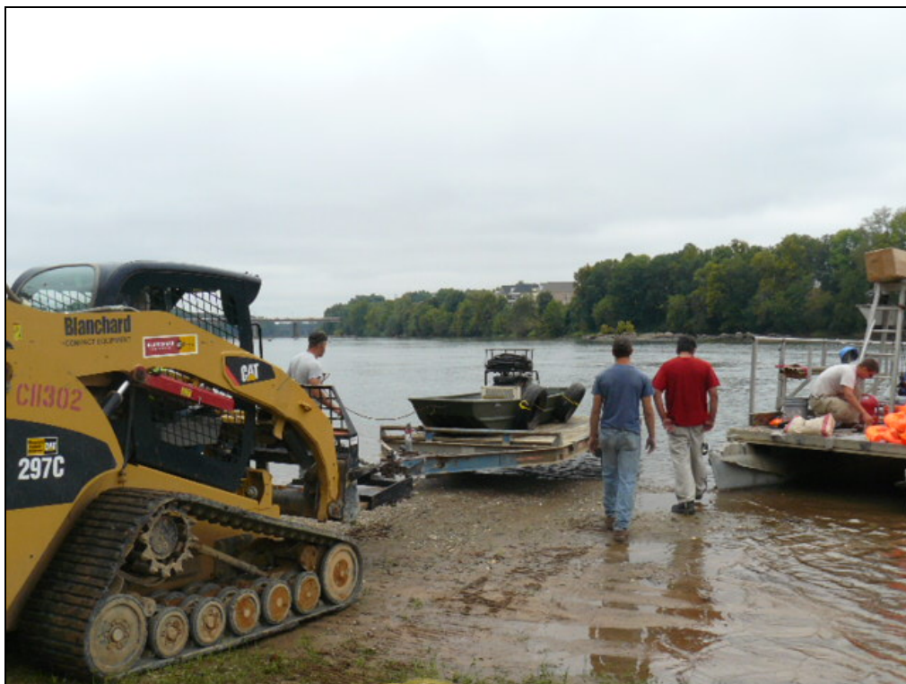
4. Preparing pontoon boat and sidecar for launch.
