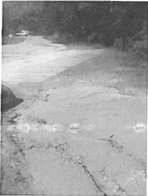
Erosion on access drive leading to dam crest.
