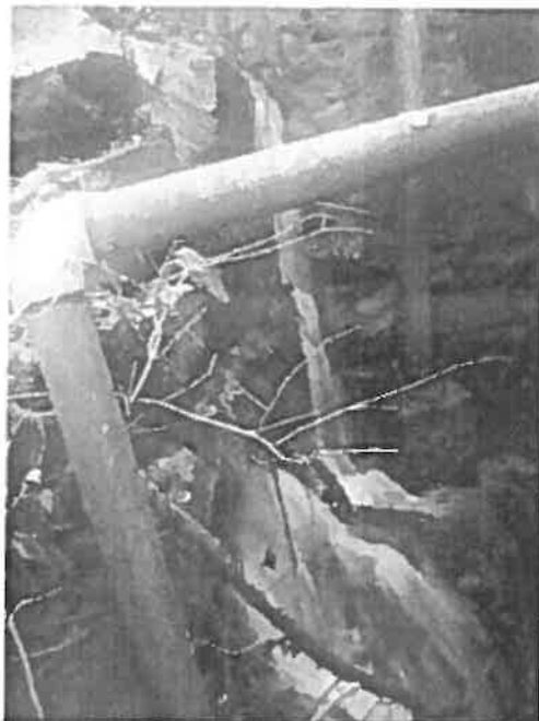
Seepage through masonry wall near penstock.
