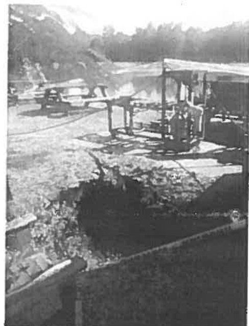
Sinkhole forming near gate for penstock.
