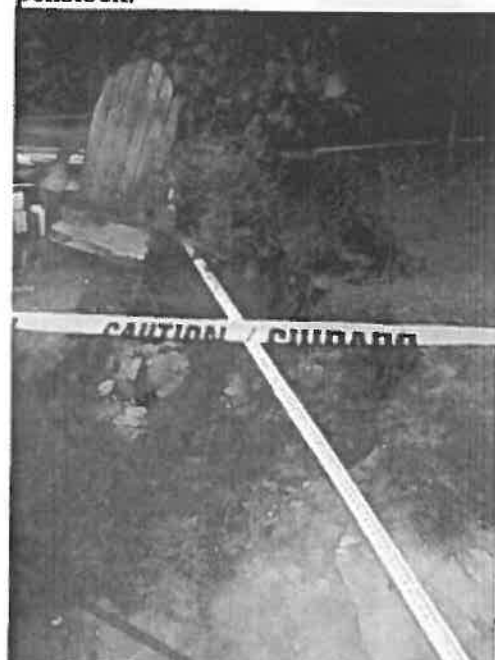
Sinkhole forming near gate for penstock.
