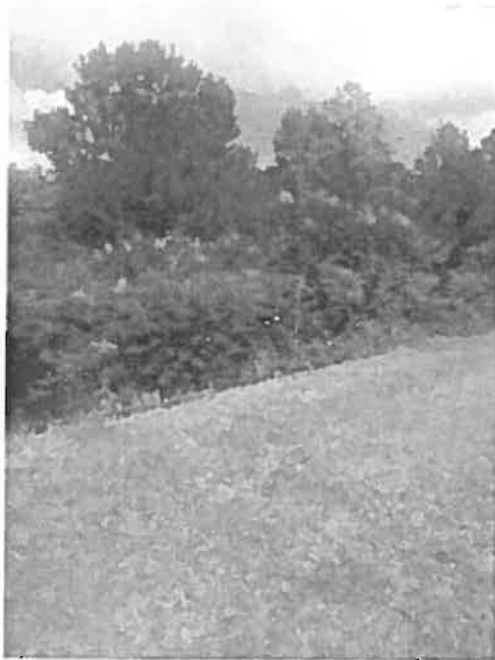
Vegetation on downstream slope of dam.
