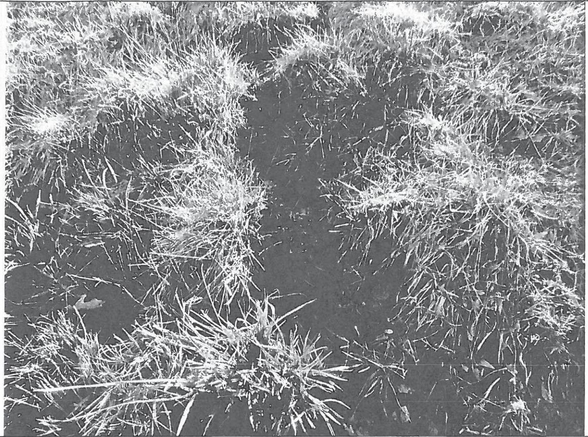
**Photo 9-** Seepage emerging from embankment on right hand side.
