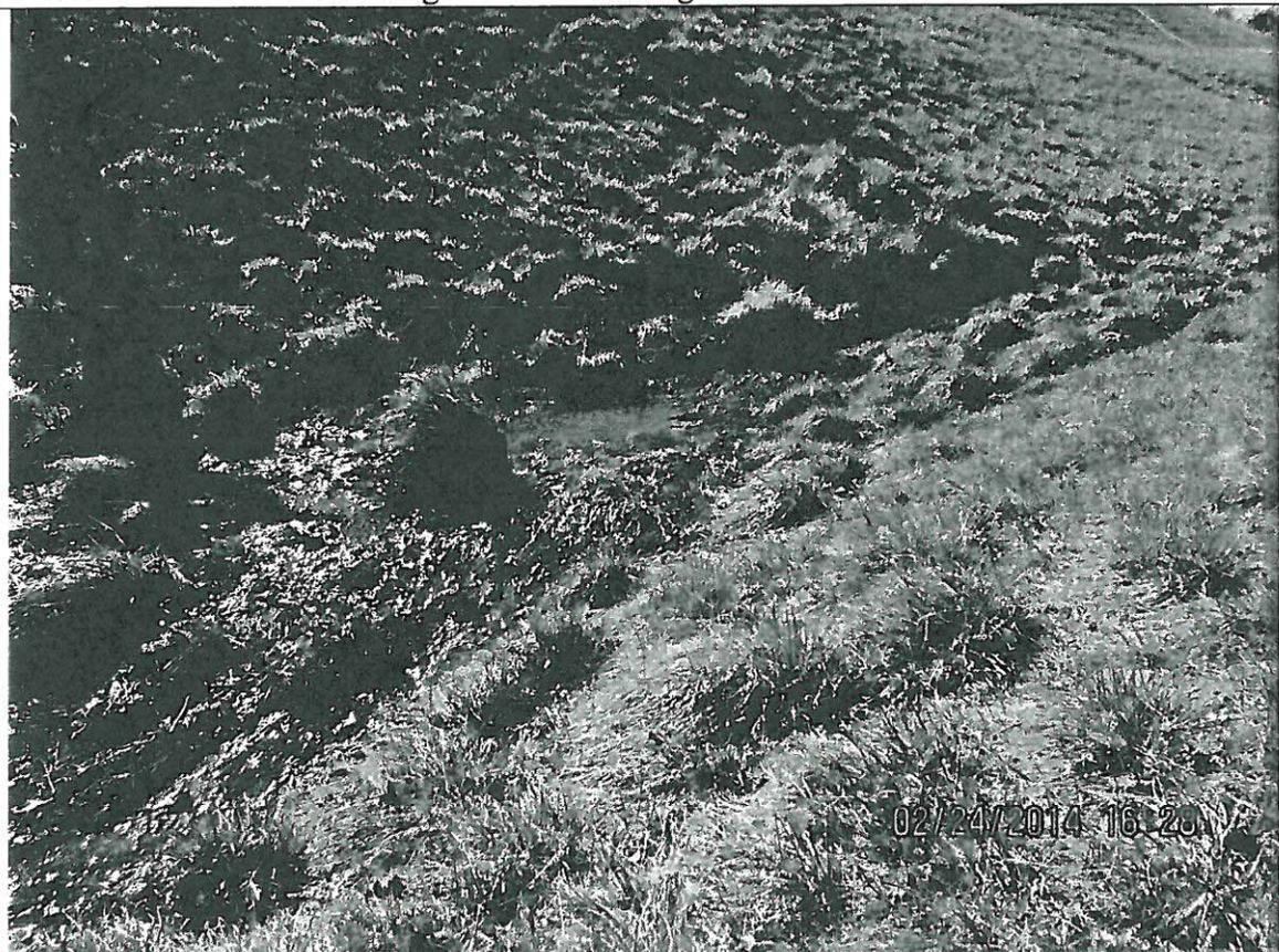
**Photo 6-** Muddy water at toe of dam on the left hand side (looking downstream) of drain.
