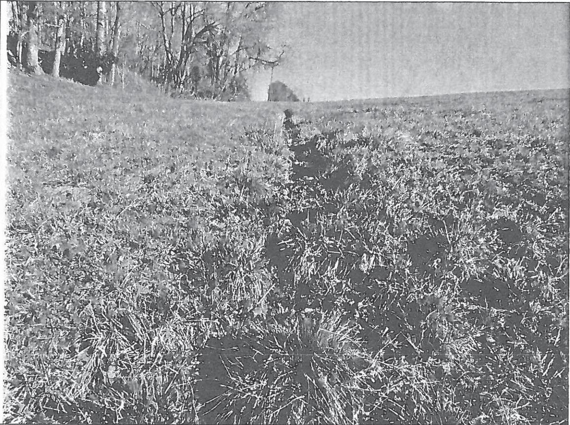
**Photo 11-** Right side groin had no flowing water. This leads to major seep in toe of dam.
