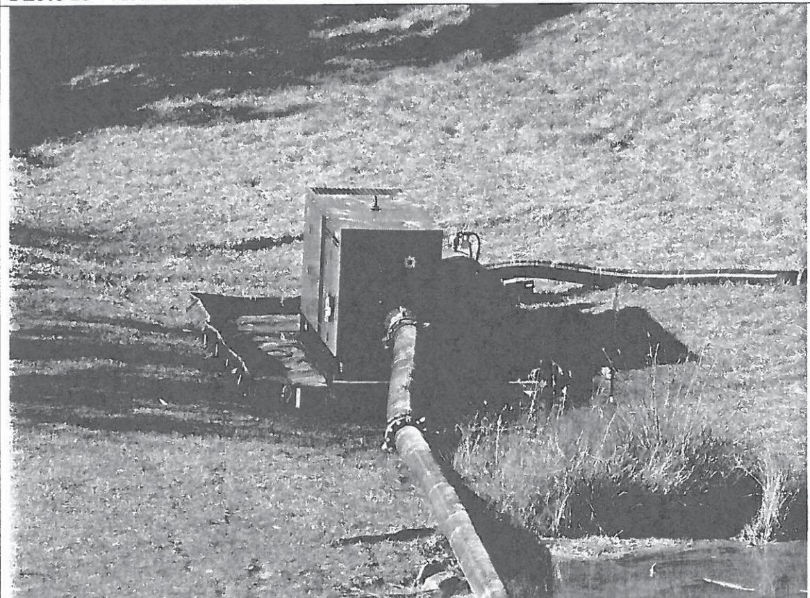
**Photo 14-** Pump in place for diverting flow around outlet pipe for slip lining.
