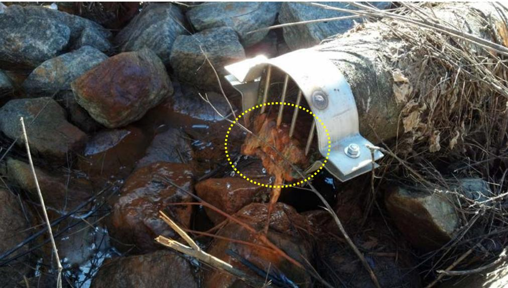
Iron Bacteria Build-Up at Toe Drains - D-2879 Huff Creek WCD Dam #2A
