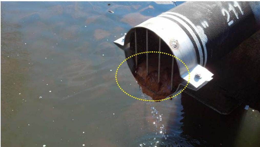
Iron Bacteria Build-Up at Toe Drains - D-2880 Huff Creek WCD Dam #3A
