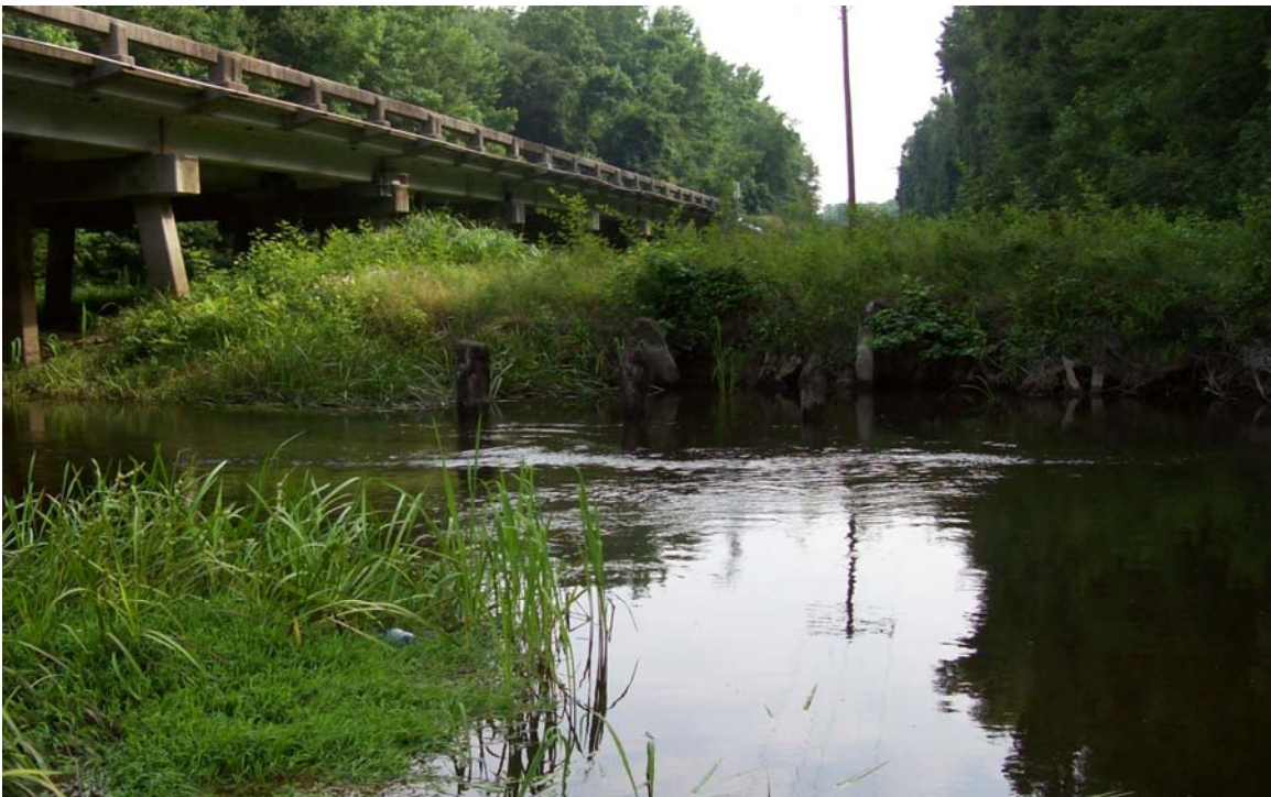
Impaired Site E-092, Hwy 3 going across
