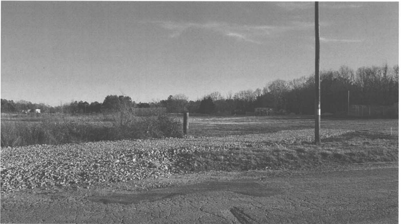
Upgraded construction entrance along Lewis Drive and frac tank in background.
