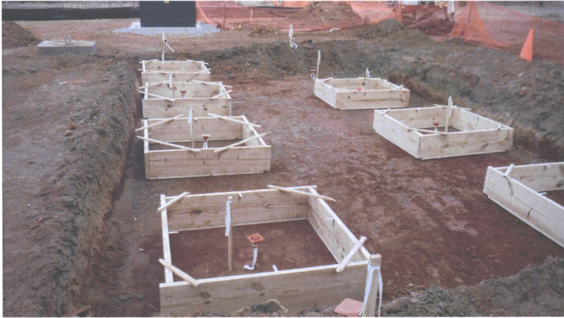
11/22/2016: Spread footer forms constructed to support the modular equipment building.
