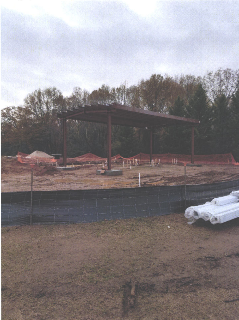
11/30/2016: Canopy frame is installed in the future equipment compound area.
